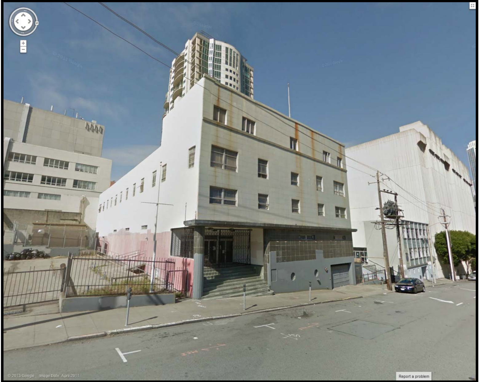
350 Fremont Street (Source: Google Maps, April 2011)
