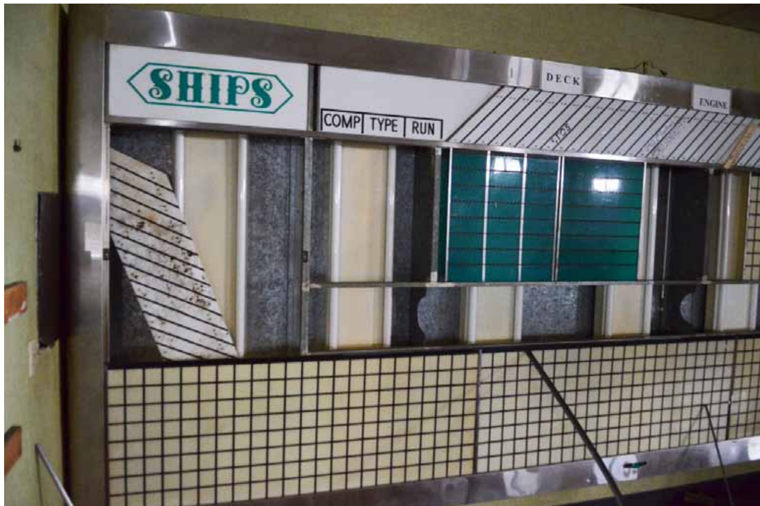
Original Job Board at existing site. Portions to be restored and incorporated as housing for Interpretive Media Display.
