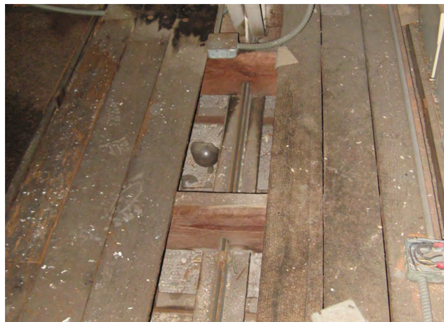
Wood walkway above flat molding of plaster grid
