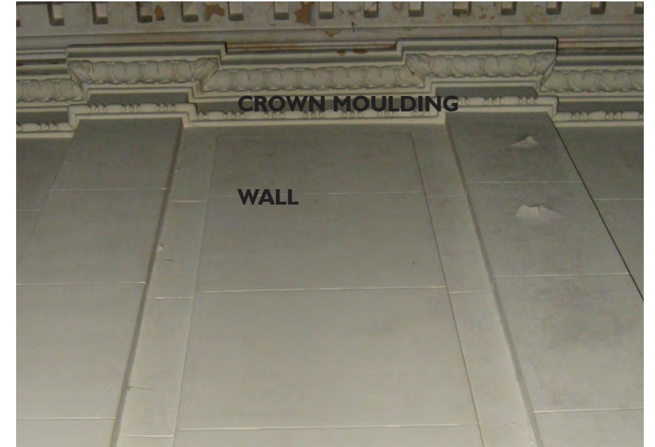
Typical Plaster Wall (Looking up at wall)
