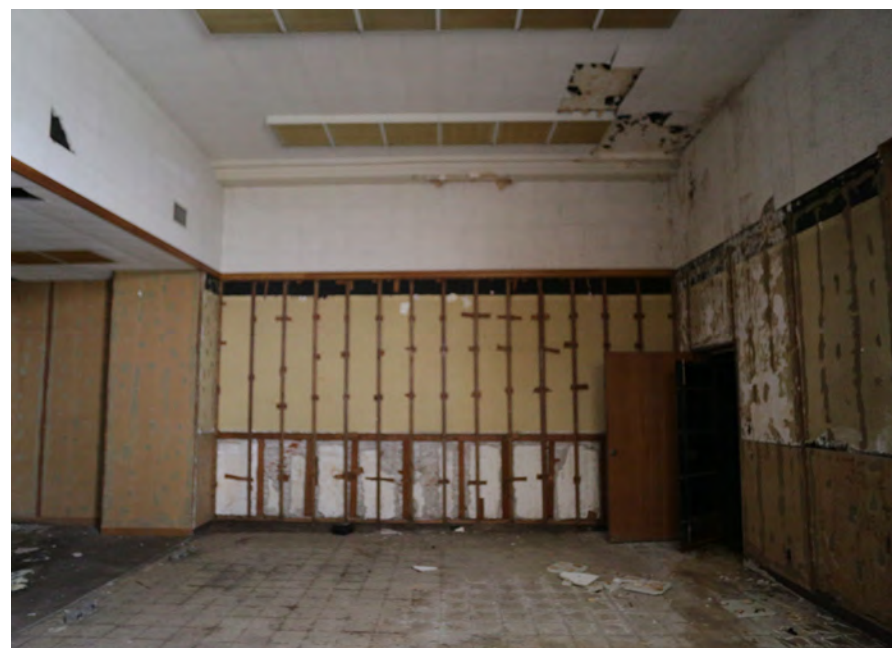
Existing condition photo of room on east side of entry hall.
