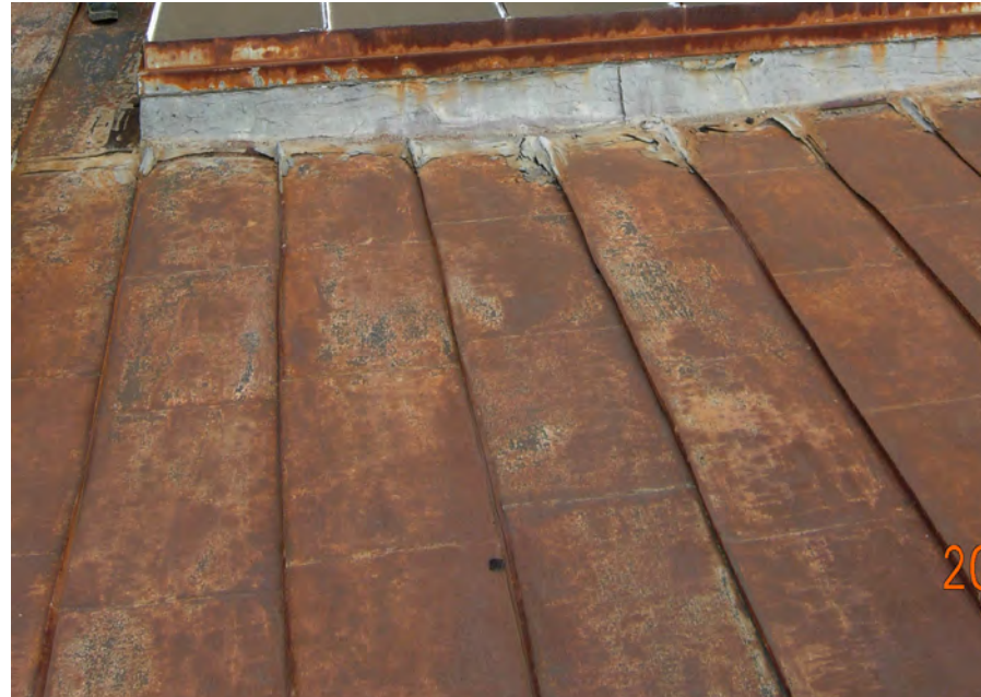
Photo showing existing roof condition
