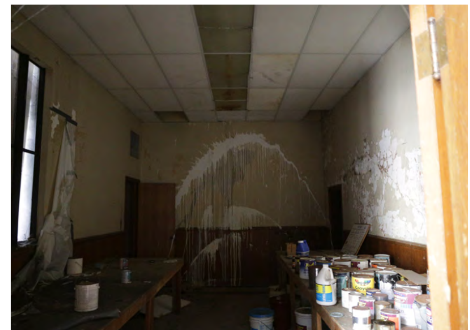
Existing condition photo of room on west side of entry hall.
