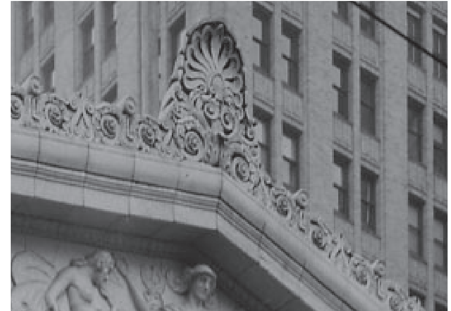
Historic photo of acroterion. ca. 1936-1964
