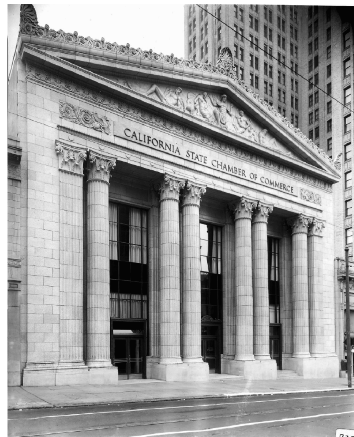
5 HISTORIC PHOTOGRAPH - SOUTH FACADE SCALE: N.T.S.
