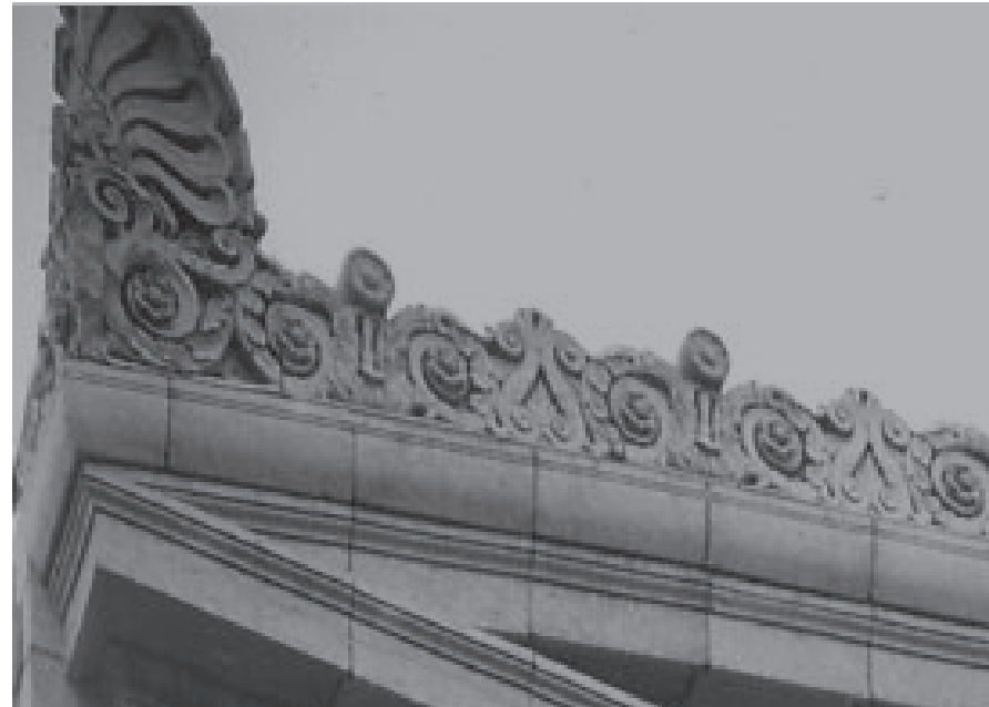
Historic photograph showing acroterion and raking pediment detail at west end of pediment. ca. 1936-1964
