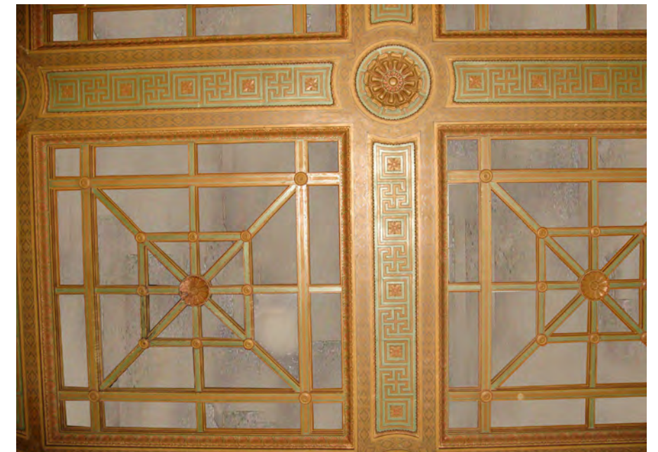
Photoshopped photograph showing proposed glazing of the laylights, which will be backlit
