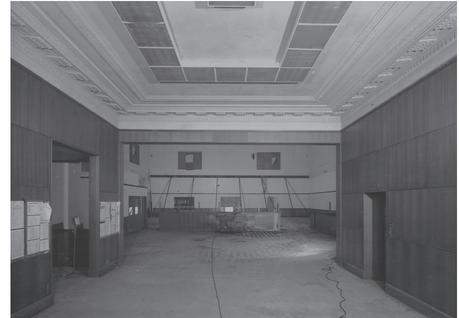
Existing condition photo of Entry Hall, looking north
