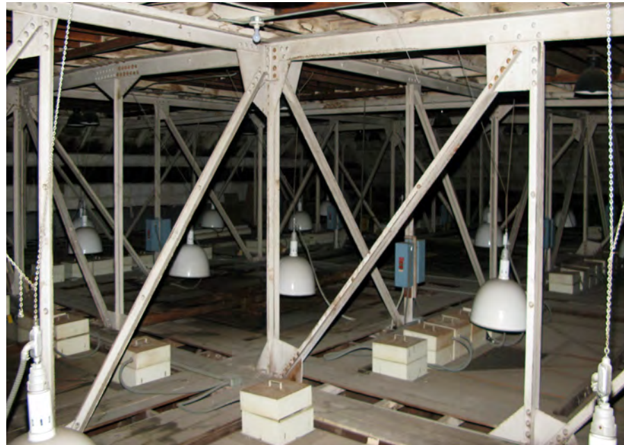
Existing riveted steel truss supporting ornamental ceiling
