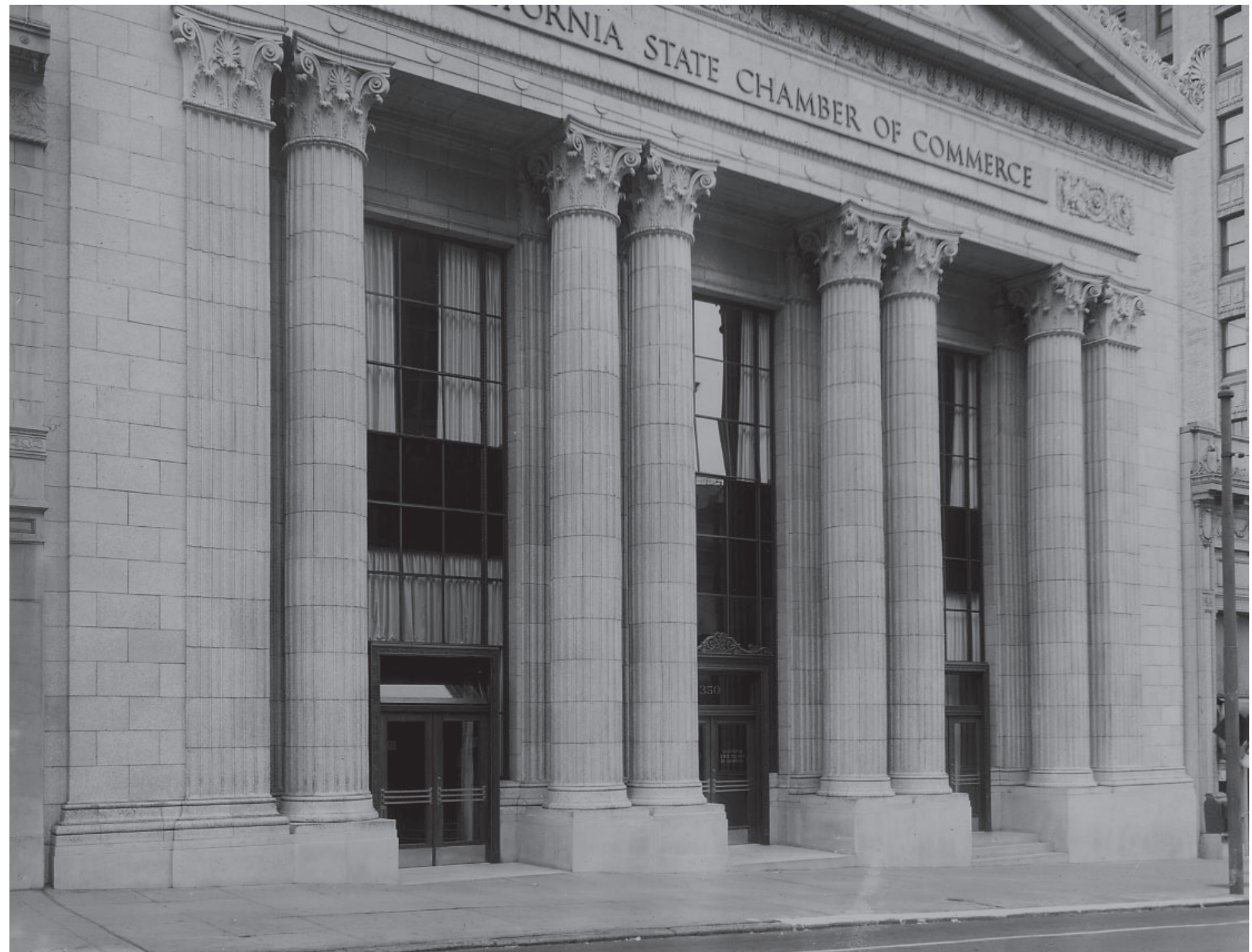
Altered condition 1928-1966 Note: Three pairs of doors and steps at center and east entry.
