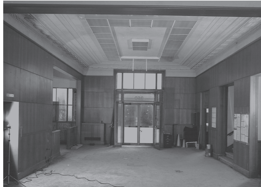
Existing condition photo of Entry Hall, looking south toward entry doors
