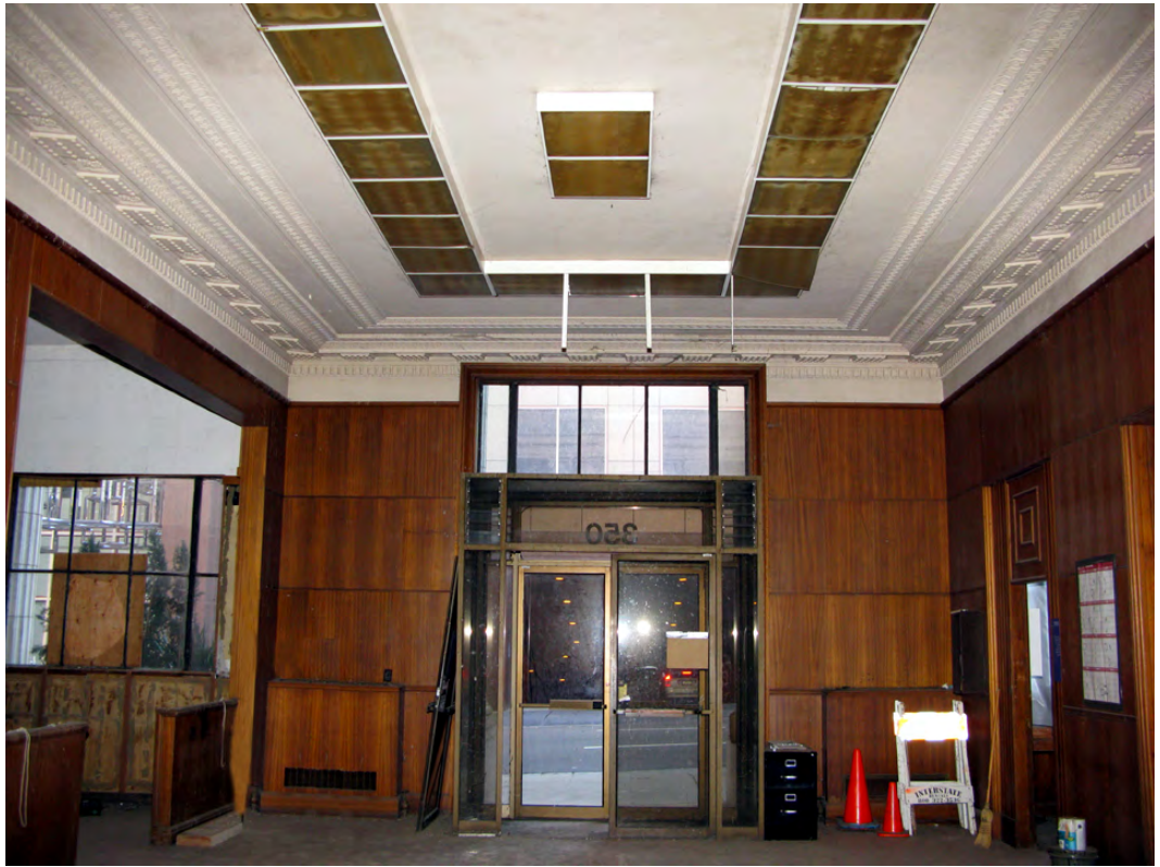
Figure 1: Main Entry of 350 Bush Street, looking south. The aluminum entrance, wood veneer paneling and fluorescent lights are non-historic features. The plaster ceiling and cornice molding are character-defining features of the building and will be retained in place.
