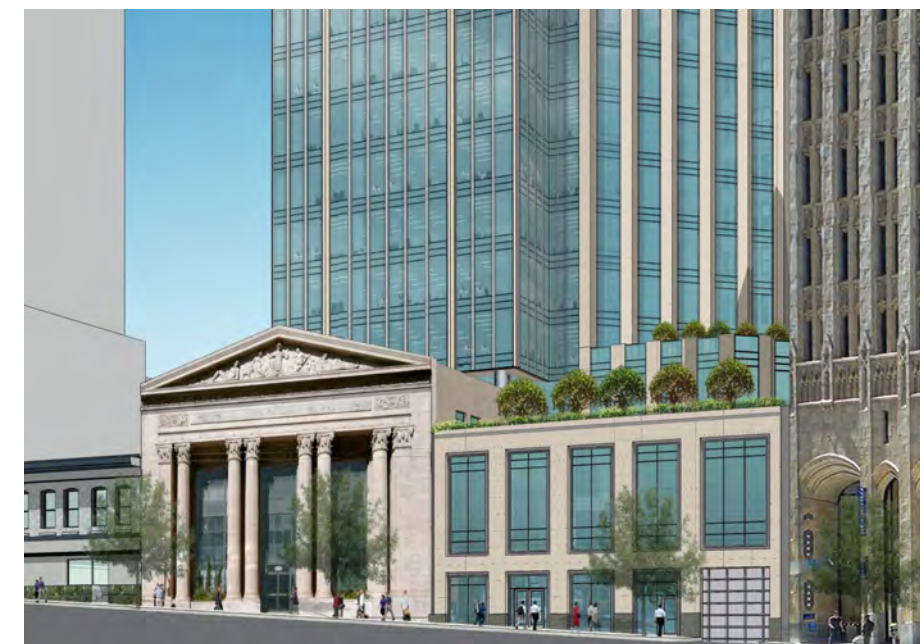
New operable windows and door to match new storefront system, an aluminum, with light silver finish.
