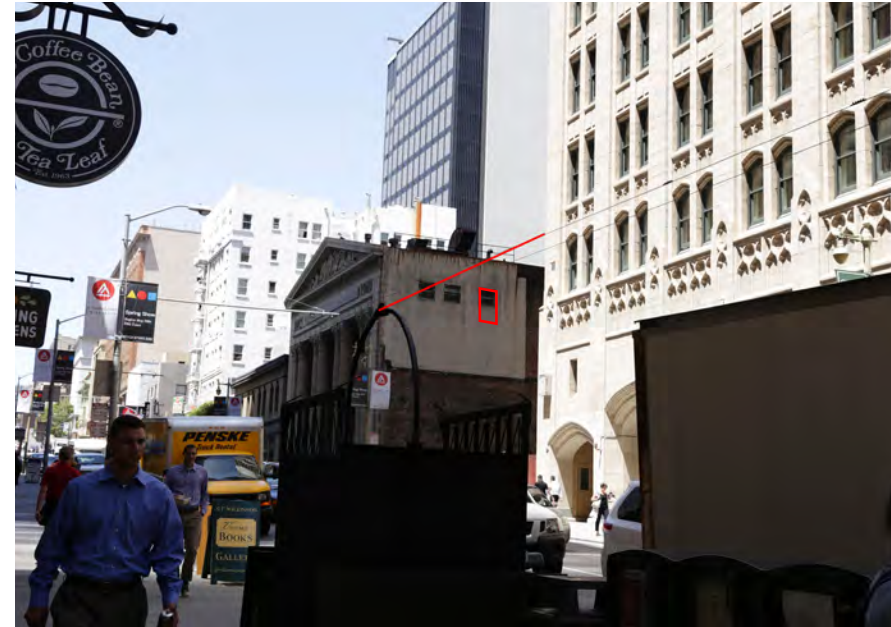
1 View Along Bush Street, looking northwest. Red line shows line of new parapet and rectangle shows window that will be replaced with a new door.
