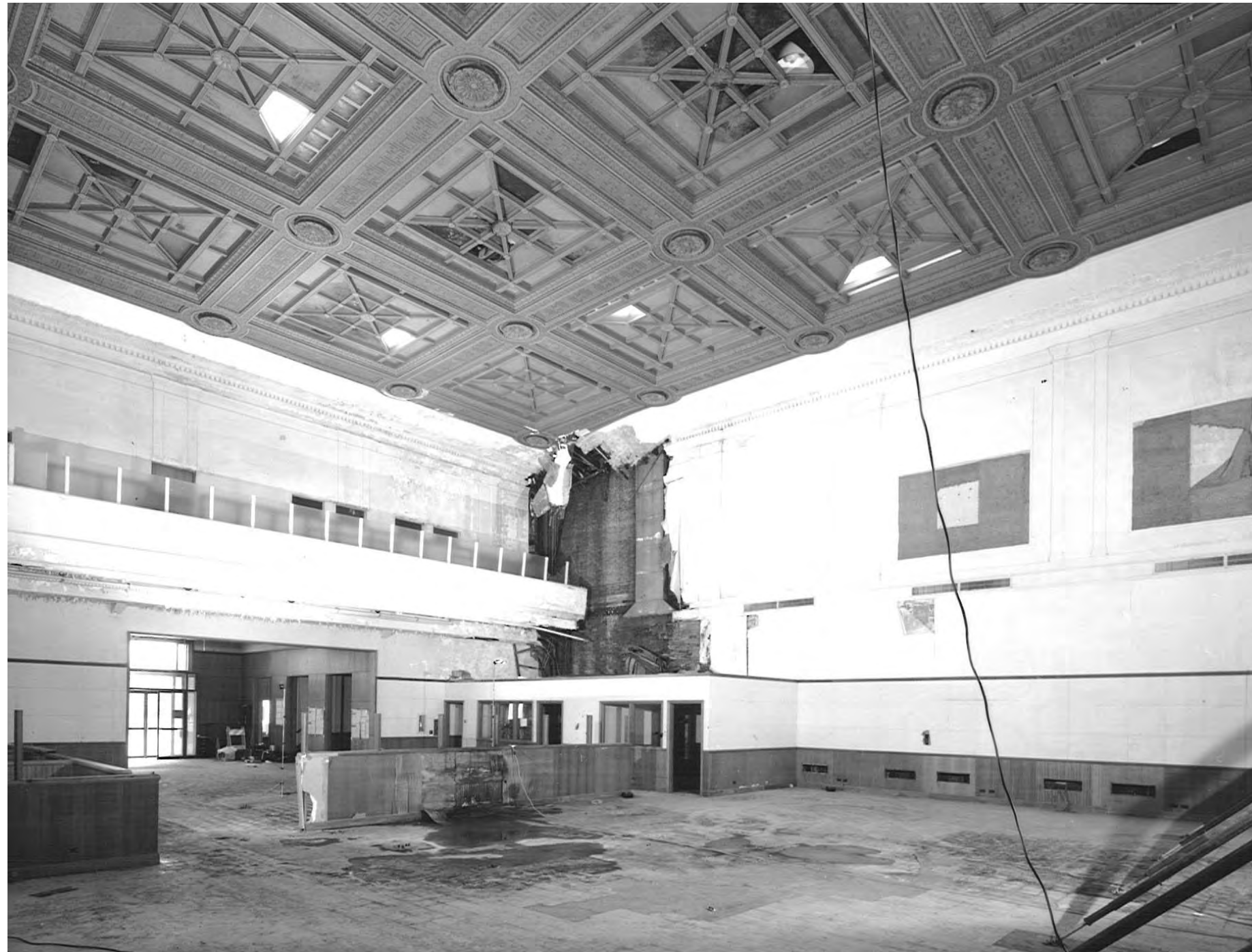
Exchange Hall looking southwest
