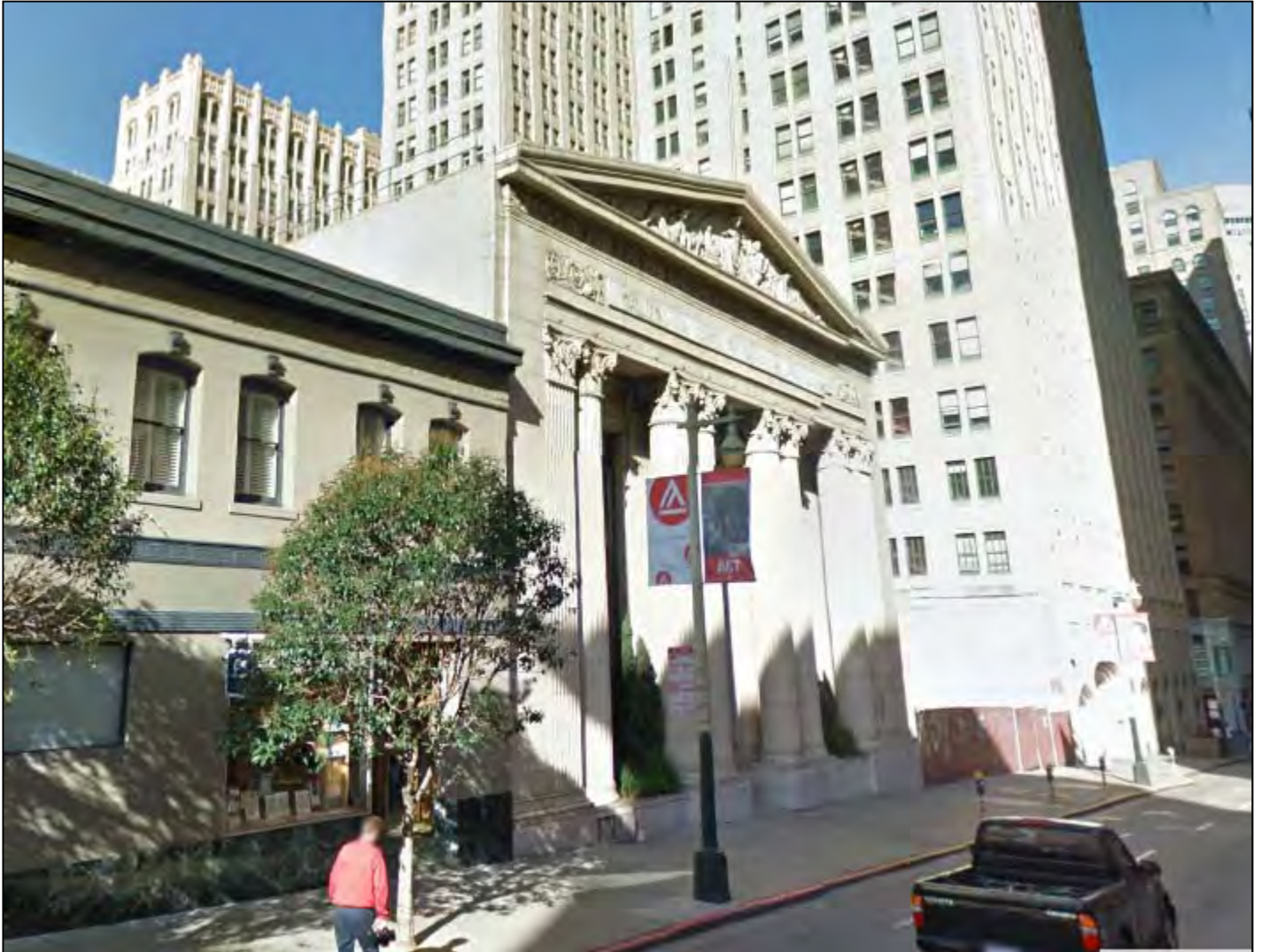
View of west elevation of 350 Bush Street from Bush Street
