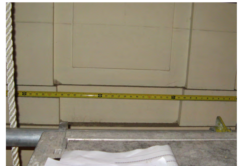
Typical Plaster Wall (Looking up at the middle of the wall)
