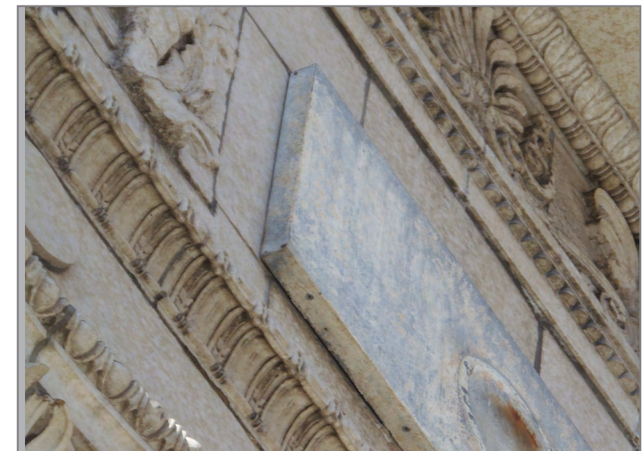
Existing signage will be removed
