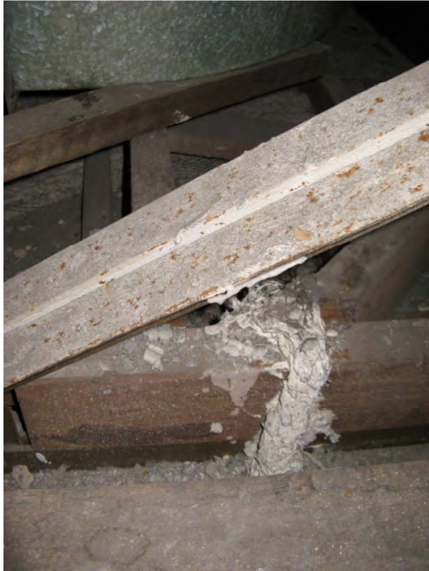
Figure 7: Exchange Hall ceiling framing showing plaster rope attached to joist.
