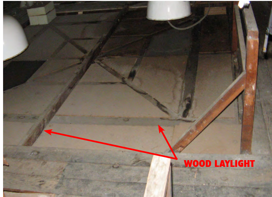
View of wood laylight from interstitial ceiling above
