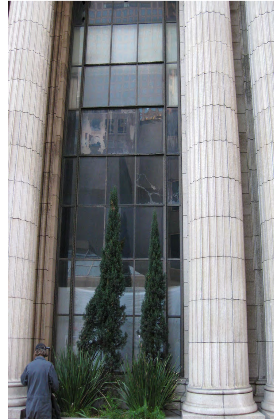
Post 1966 and current condition today. Note: Side doors removed, planters added and windows enlarged.
