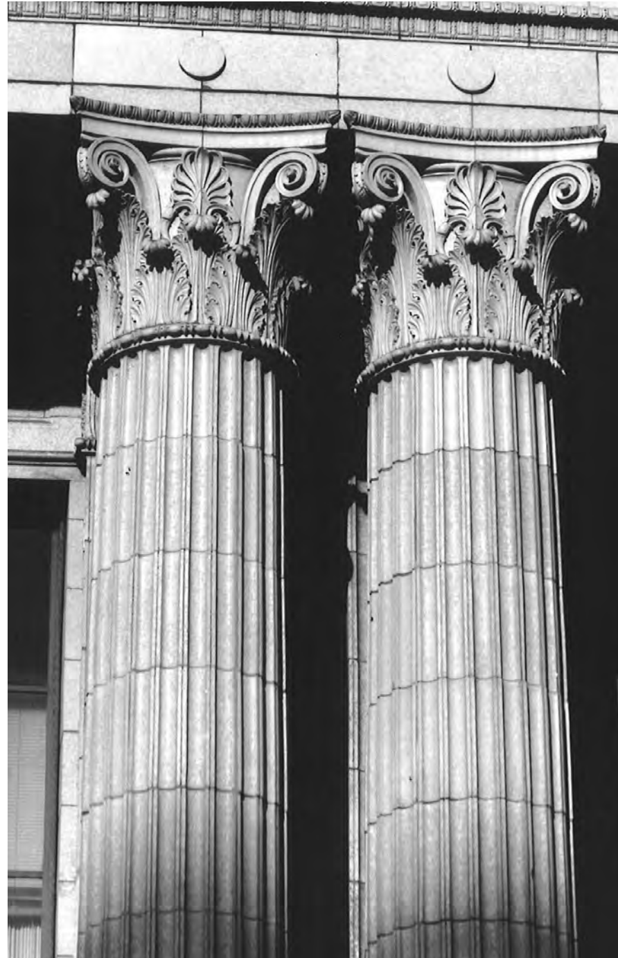
Double columns at Bush Street facade (William Porter)
