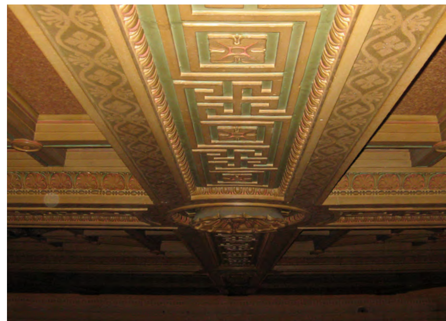
Close up view of plaster detail at ceiling
