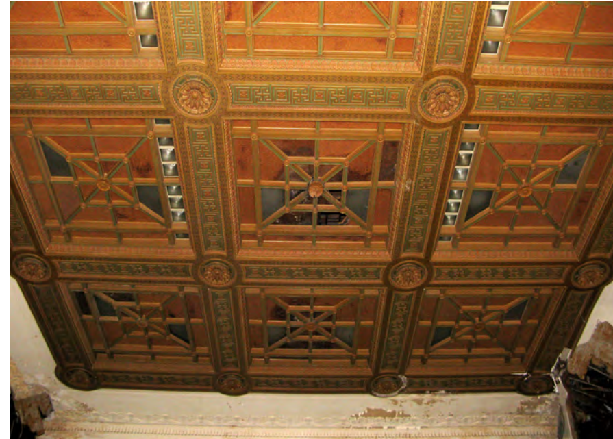
Existing coffered ceiling features decorative plaster and wood laylights
