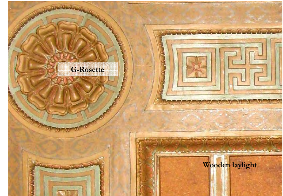
Polychromatic plaster and wood ceiling components
