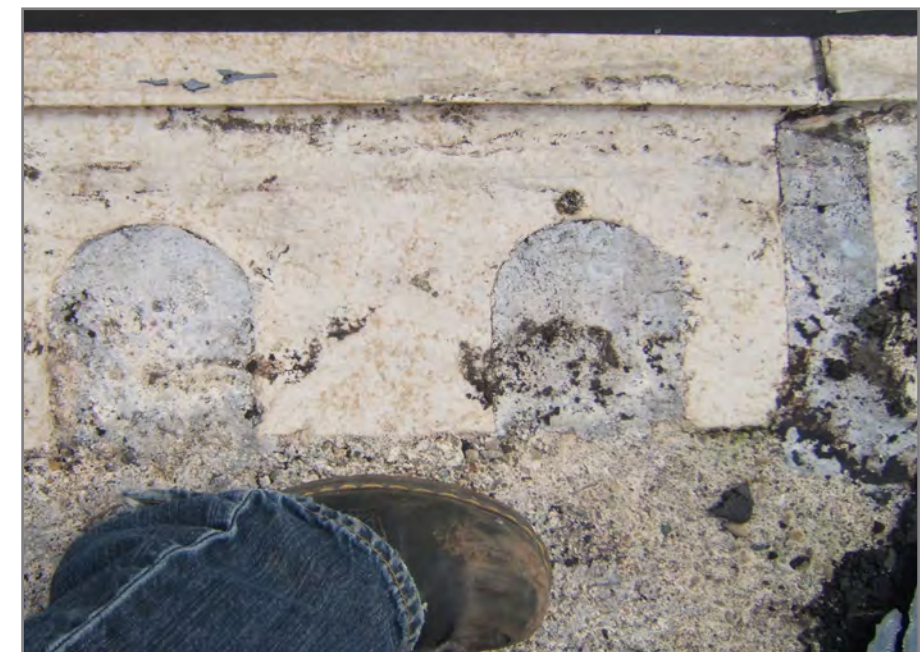
Existing photograph showing the top of the terra cotta raking cornice. The acroteria would have attached to the cornice.
