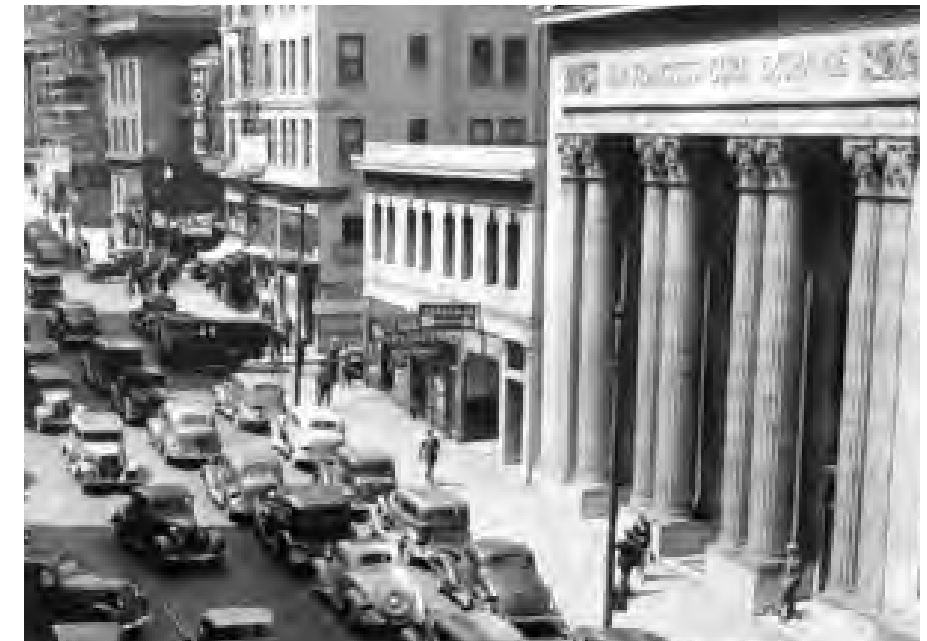
View along Bush Street, looking northwest, 1937 (San Francisco Public Library)
