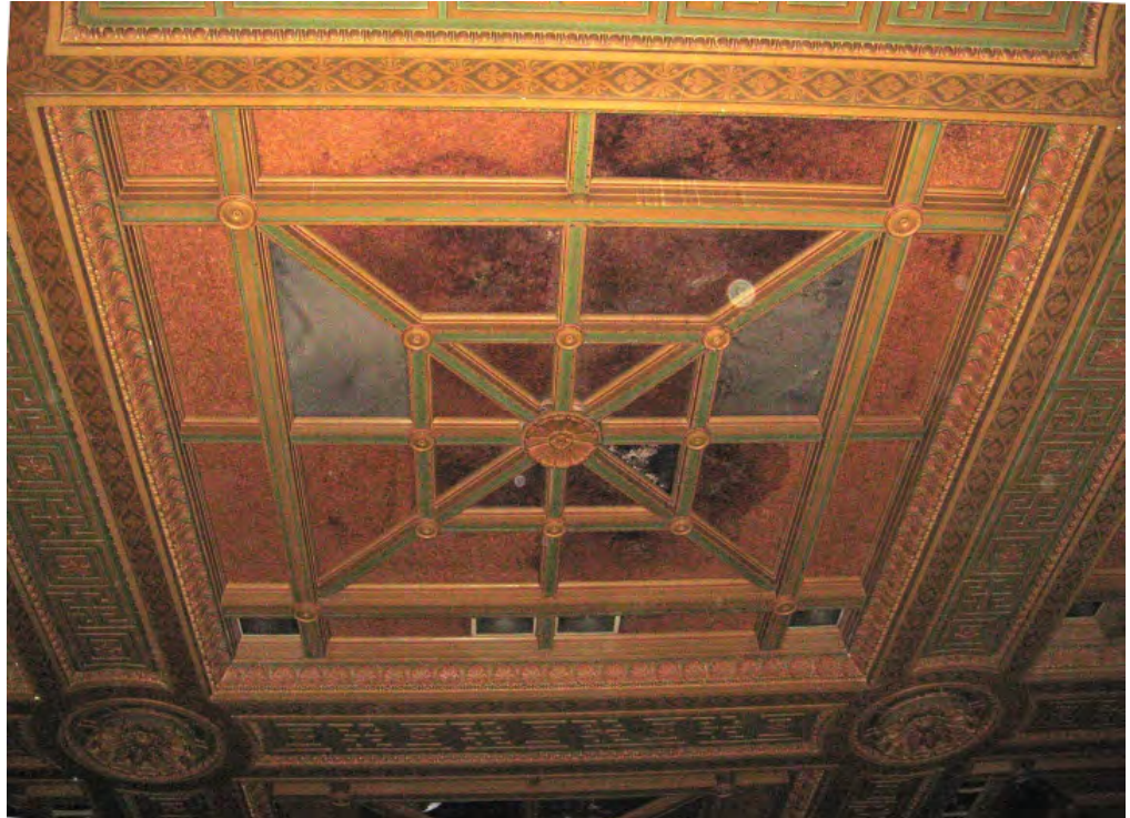
Figure 4: 350 Bush St., Exchange Hall ceiling, showing typical panel of historic laylight and surrounding architectural details, including paneled beams with acanthus leaf molding and rosettes.
