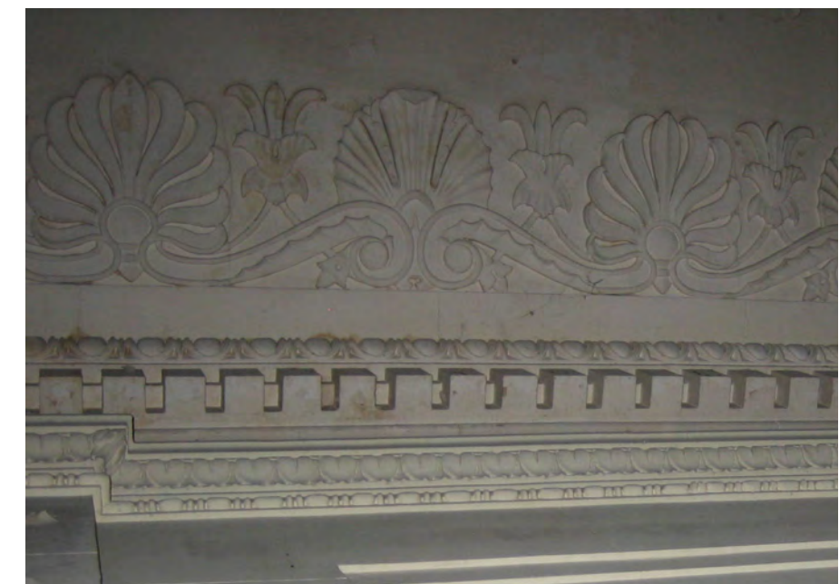
Existing plaster crown molding
