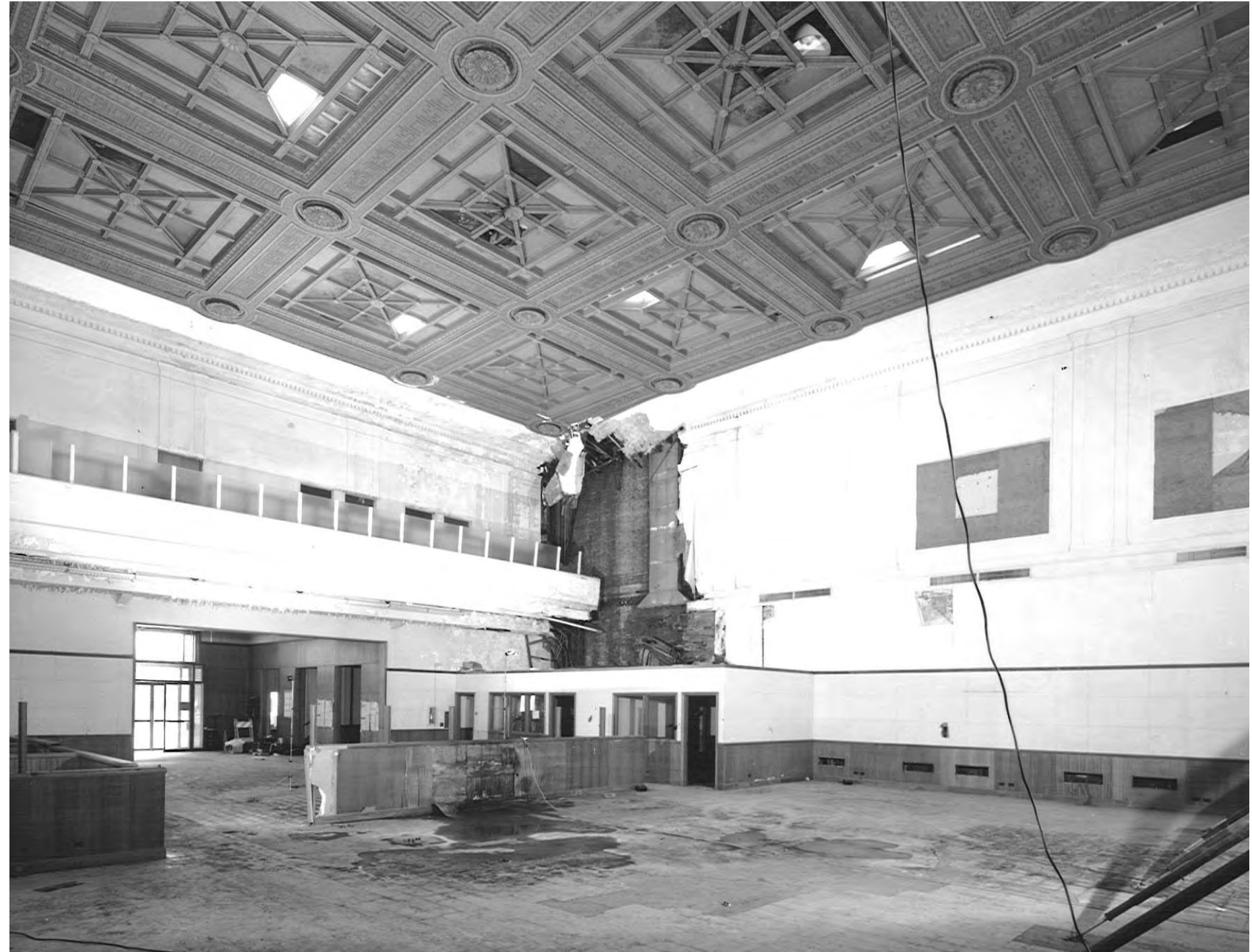
The existing condition of the Exchange Hall floor.
