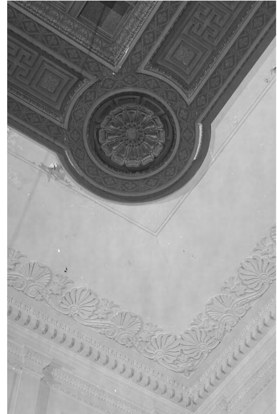
Interior showing plaster ceiling and wood laylight detail in Mining Exchange Hall (William Porter)
