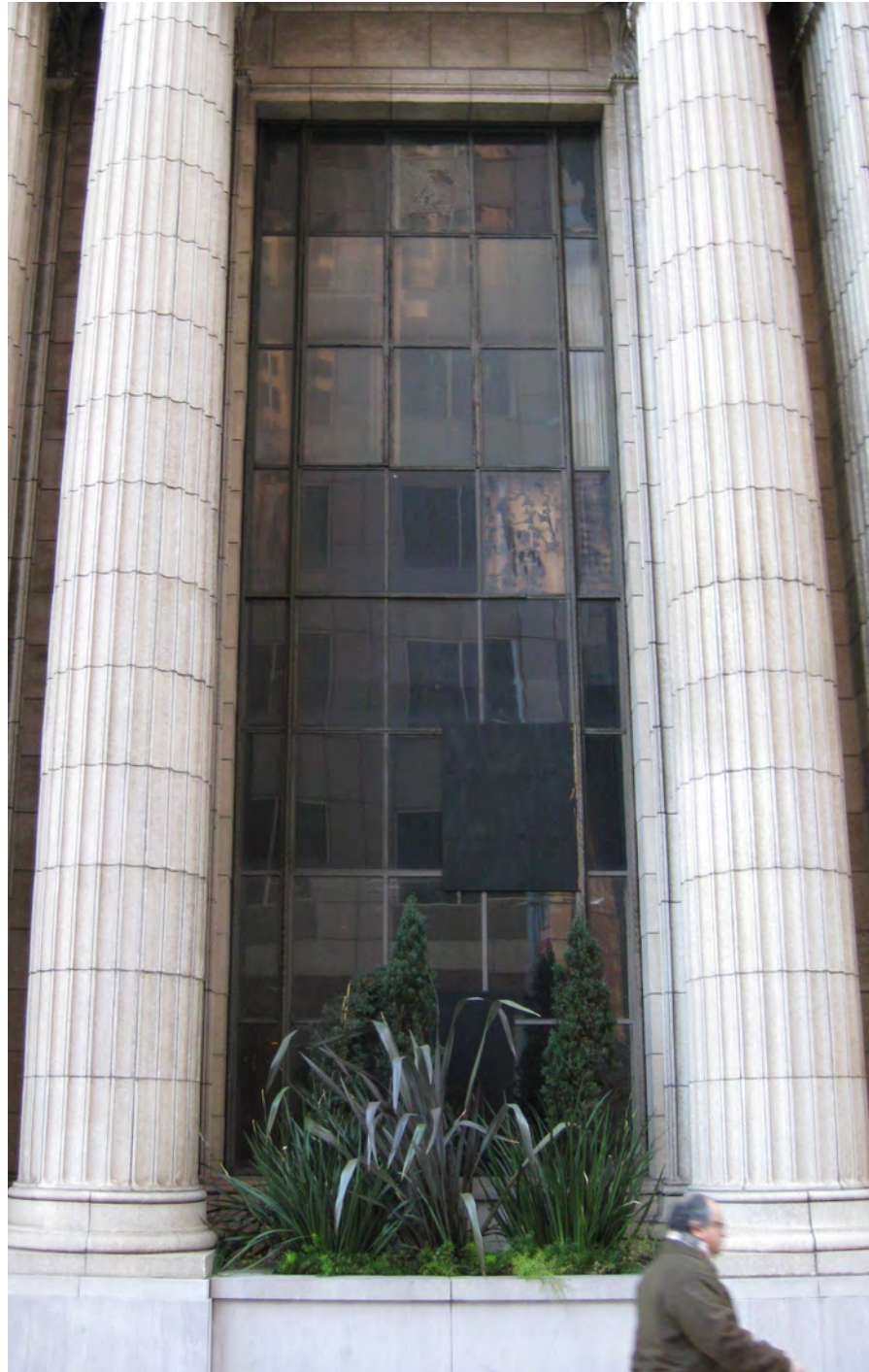
Post 1966 and current condition today. Note: Side doors removed, planters added and windows enlarged.
