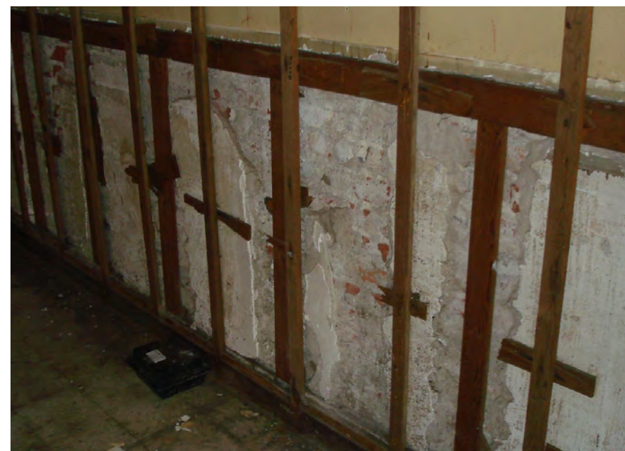
Wall furring and non historic materials.
