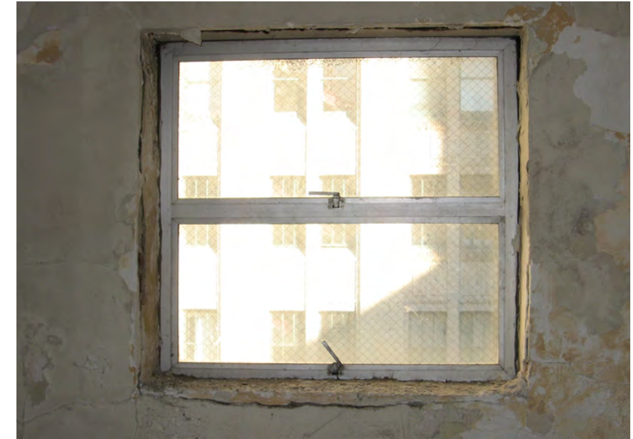
Non-historic windows at the east facade
