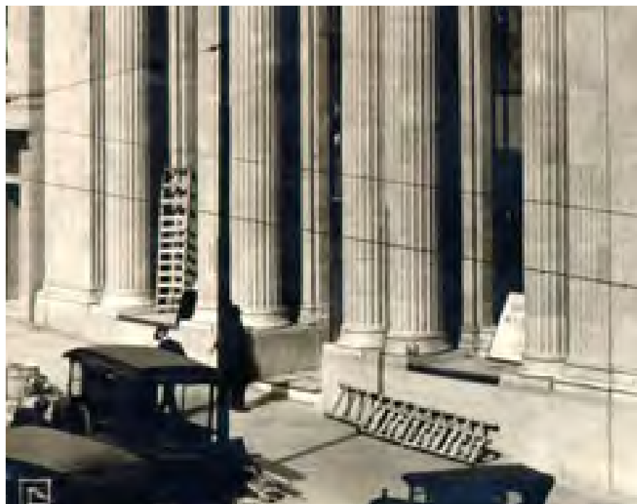
Original condition. Note: Single pair of doors between columns at center of building.
