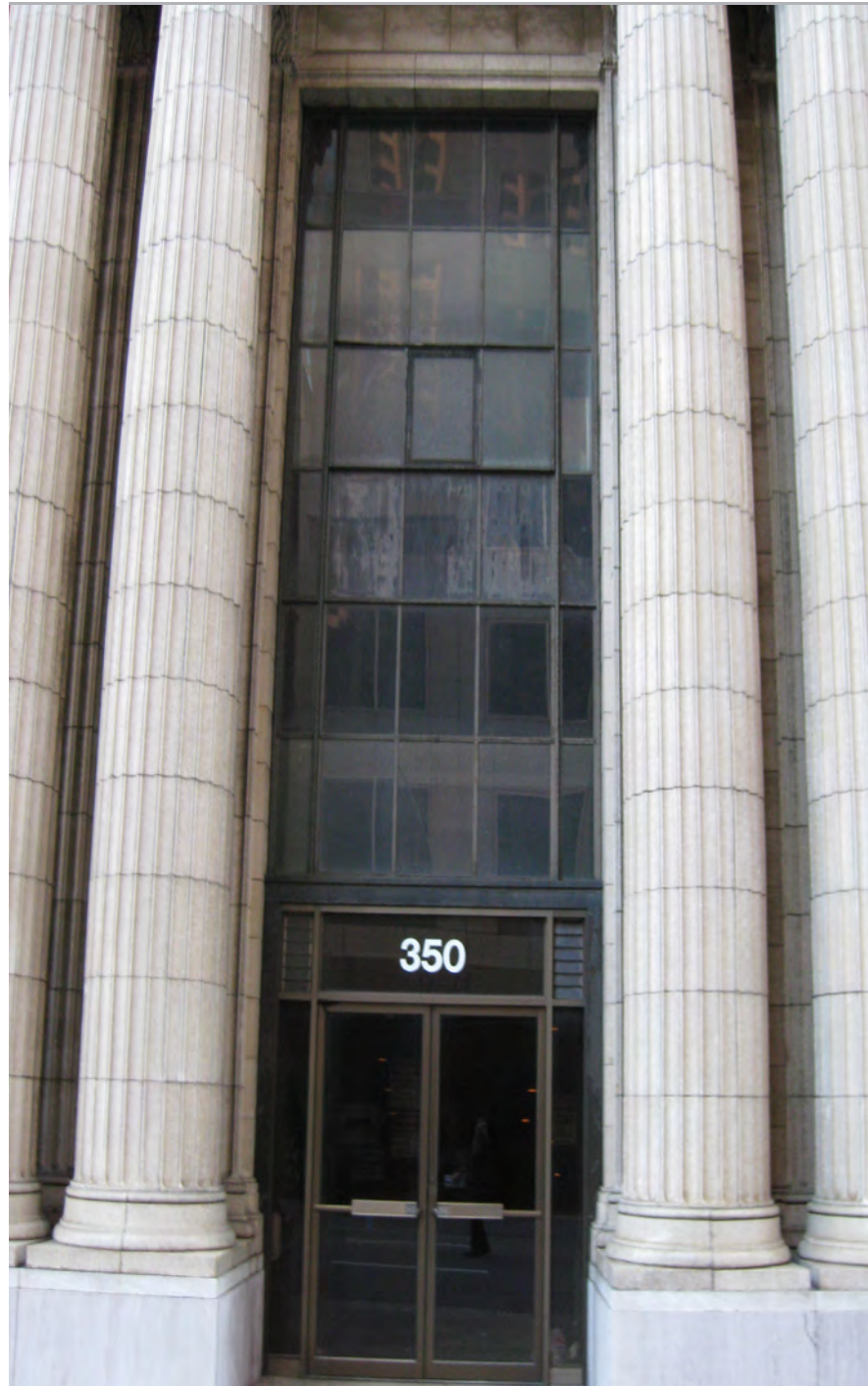
Post 1966 and current condition today. Note: Replacement aluminum storefront with sidelight jalousie windows.
