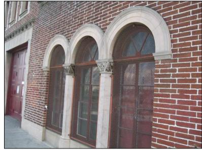
**Photograph 5**: cast stone elements and detailing at window arches and pilasters, camera facing east, 3/5/2009.
