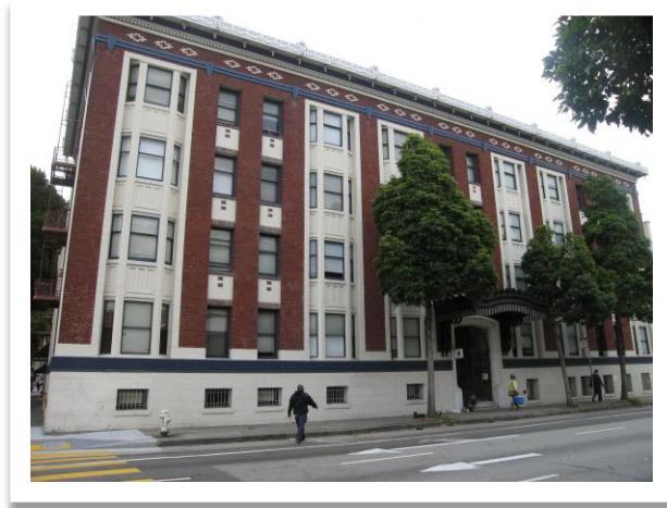
Photo: 150 Franklin Street building, part of the Market Street Masonry Landmark District.
