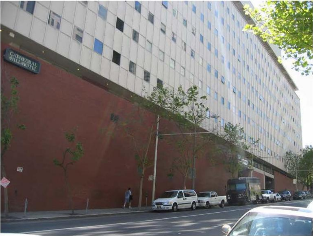
View looking southwest from Post Street
