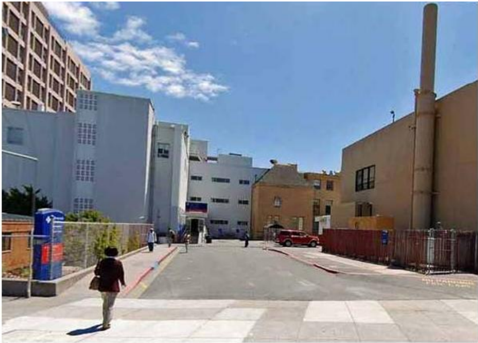
View looking east from San Jose Avenue
