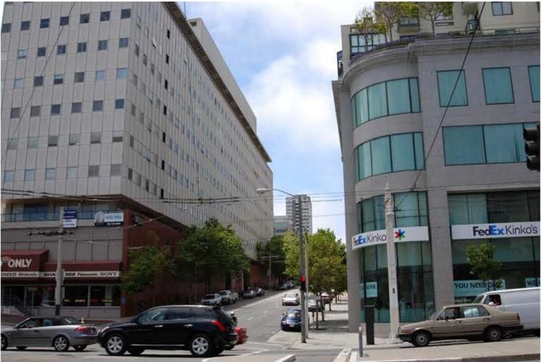
View looking southwest from Van Ness Avenue and Post Street
