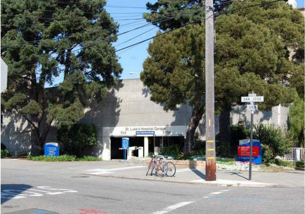
Duncan St. Parking Garage: View looking northeast from Duncan Street and San Jose Avenue
