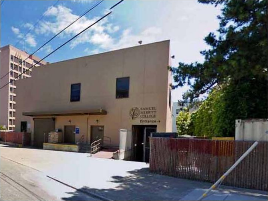
Hartzell Building: View looking east from San Jose Avenue
