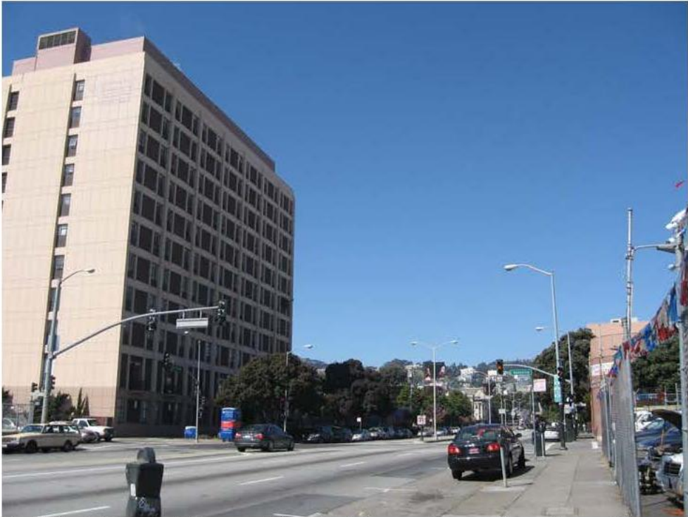
St. Luke's Hospital Tower: View looking southwest from Cesar Chavez Street
