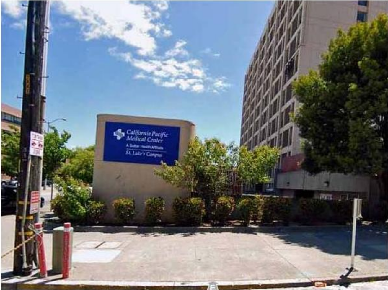
St. Luke's Hospital Tower: View looking east from San Jose Avenue
