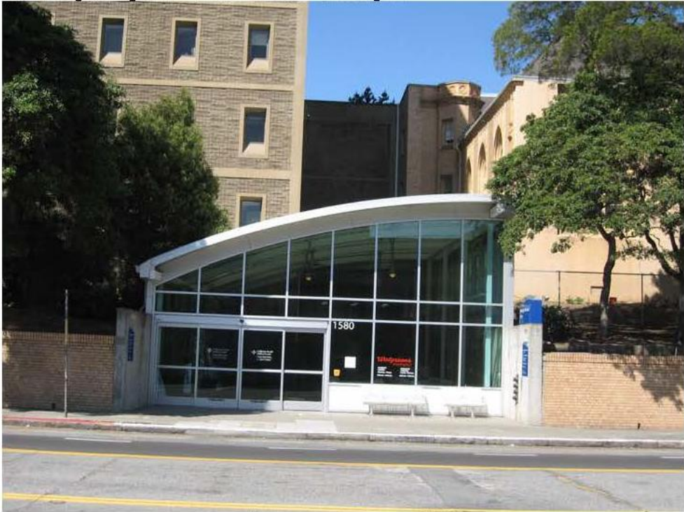
Entrance to Monteagle Building and 1912 Building: View looking west from Valencia Street
