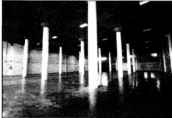
INTERIOR VIEW OF TENANT'S SPACE (CURRENT)
