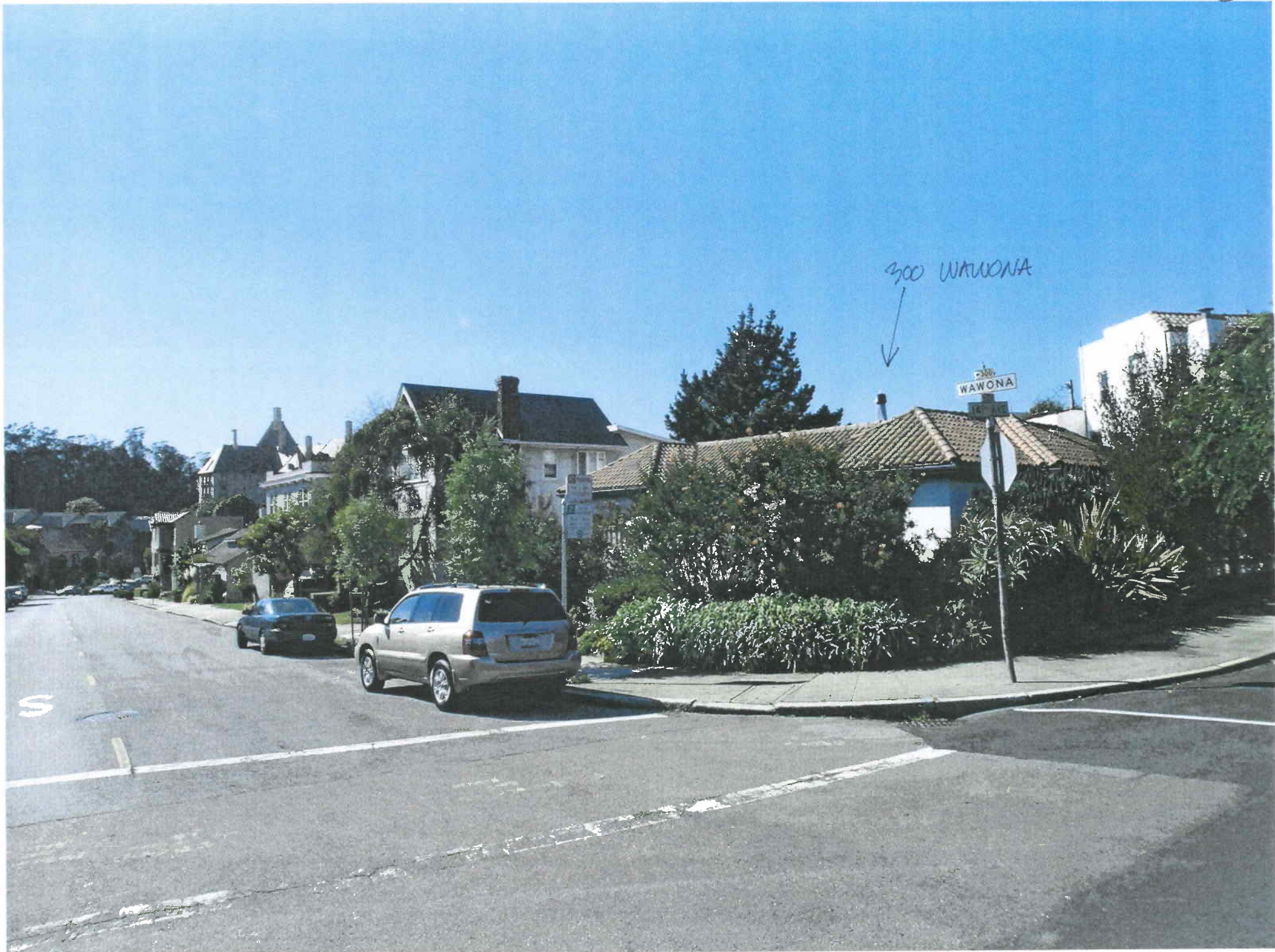
PROJECT AT 300 WAWONA AS SEEN FROM CORNER INTERSECTION
