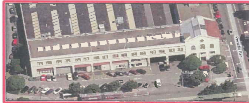
Existing Conditions on North Side of Geary Blvd. (Opposite City Center)
