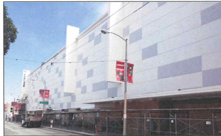
View of Existing Conditions Looking East Along Geary Blvd.
