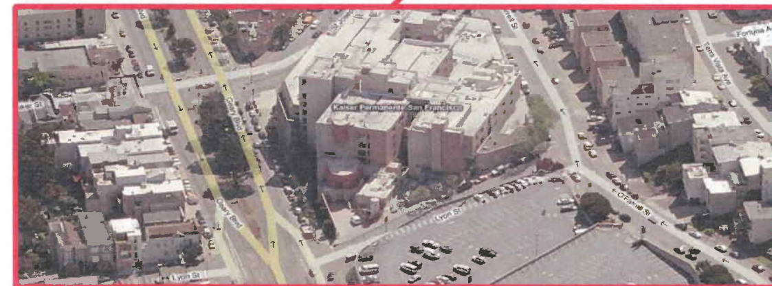
Existing Conditions on East Side of Lyon Street (Opposite City Center)
