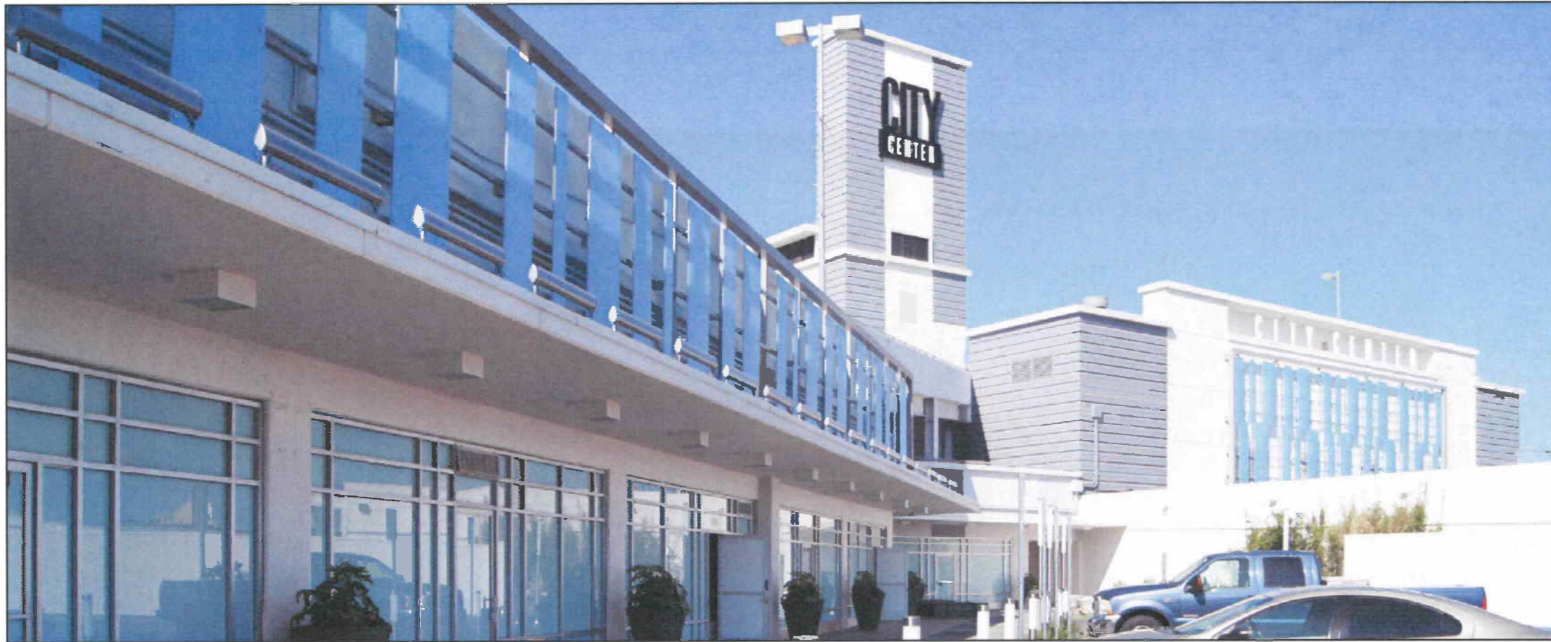
View of Existing Conditions Looking Northwest Toward Building at Parking Lot E. Proposed location for the following CUP tenancy: Panera Bread, Chipotle Mexican Grill, GNC
