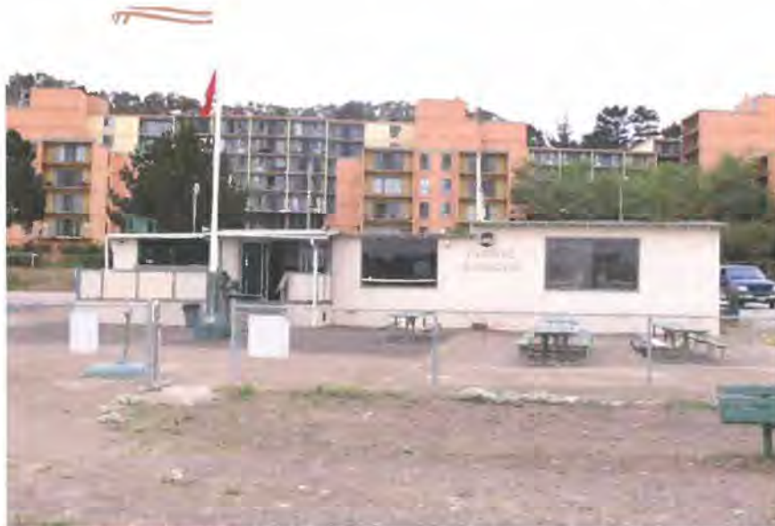
Figure 22. Northeast façade of the Club house, viewed facing southwest Source: Page & Turnbull, 2013
