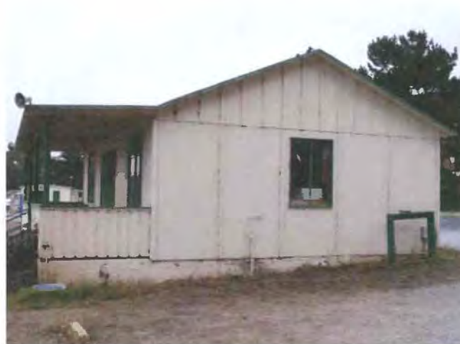
Figure 35. Northwest façade, viewed facing southeast Source: Page & Turnbull, 2013
