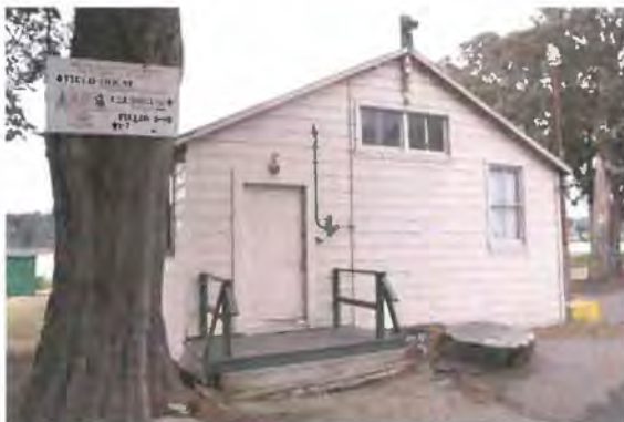
Figure 39. Southeast façade. Source: Page & Turnbull, 2013
