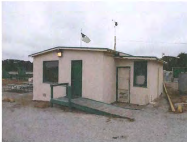
Figure 27. Northwest façade, viewed facing southeast. Source: Page & Turnbull, 2013
