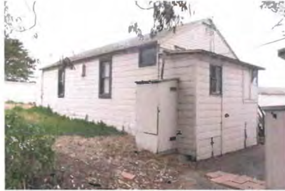
Figure 51. South and east facades, viewed facing northwest Source: Page & Turnbull, 2013
