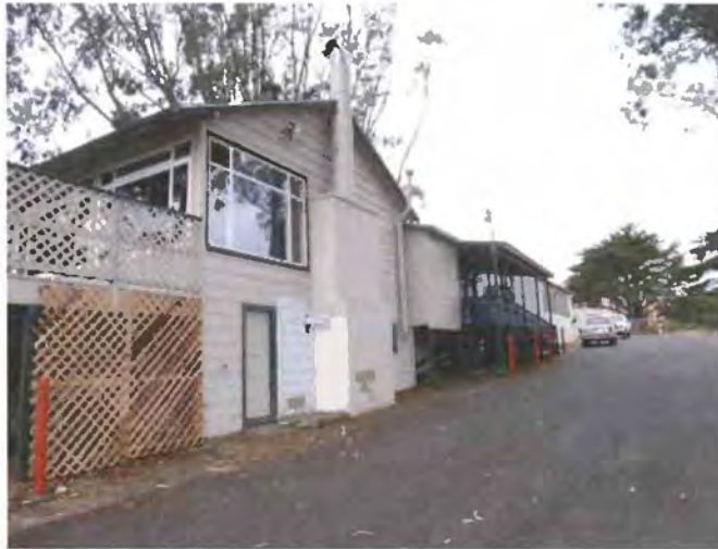
Figure 56. North façade, viewed facing southwest. Source: Page & Turnbull, 2013
