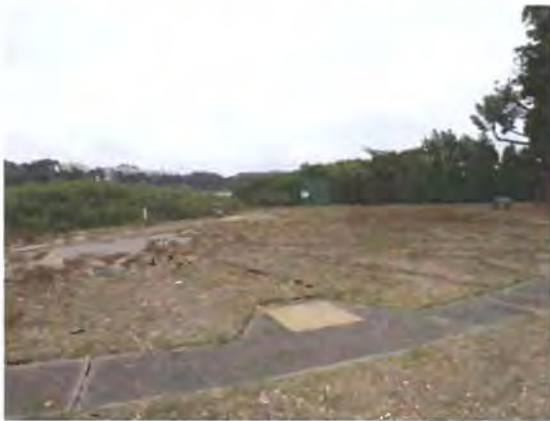
Figure 13. Shooting station on the arc of Field 9. Source: Page & Turnbull, 2013
