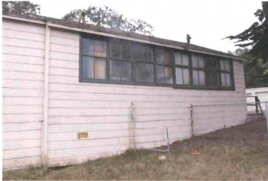
Figure 45. Detail of windows on northwest façade. Source: Page & Turnbull, 2013
