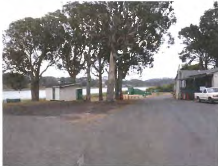
Figure 12. Automobile access drive, viewed facing southeast toward Fields 8 and 9 Source: Page & Turnbull, 2013
