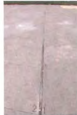
Figure 16. Distance marks on concrete apron of skeet field Source: Page & Turnbull, 2013
