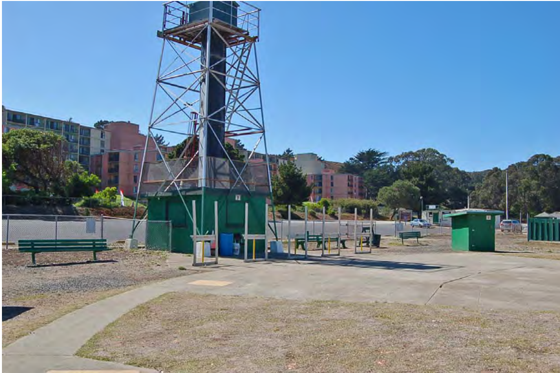
Photo 18. Duck Tower, Five Stand frames, and a Fire Stand equipment shed on Field 6; view to W (D. Bradley, September 2013)
