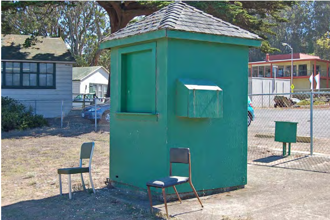
Photo 14. Skeet equipment shed on Field 7 (typical example of feature found on Fields 4 to 7); view to S (D. Bradley, September 2013).
