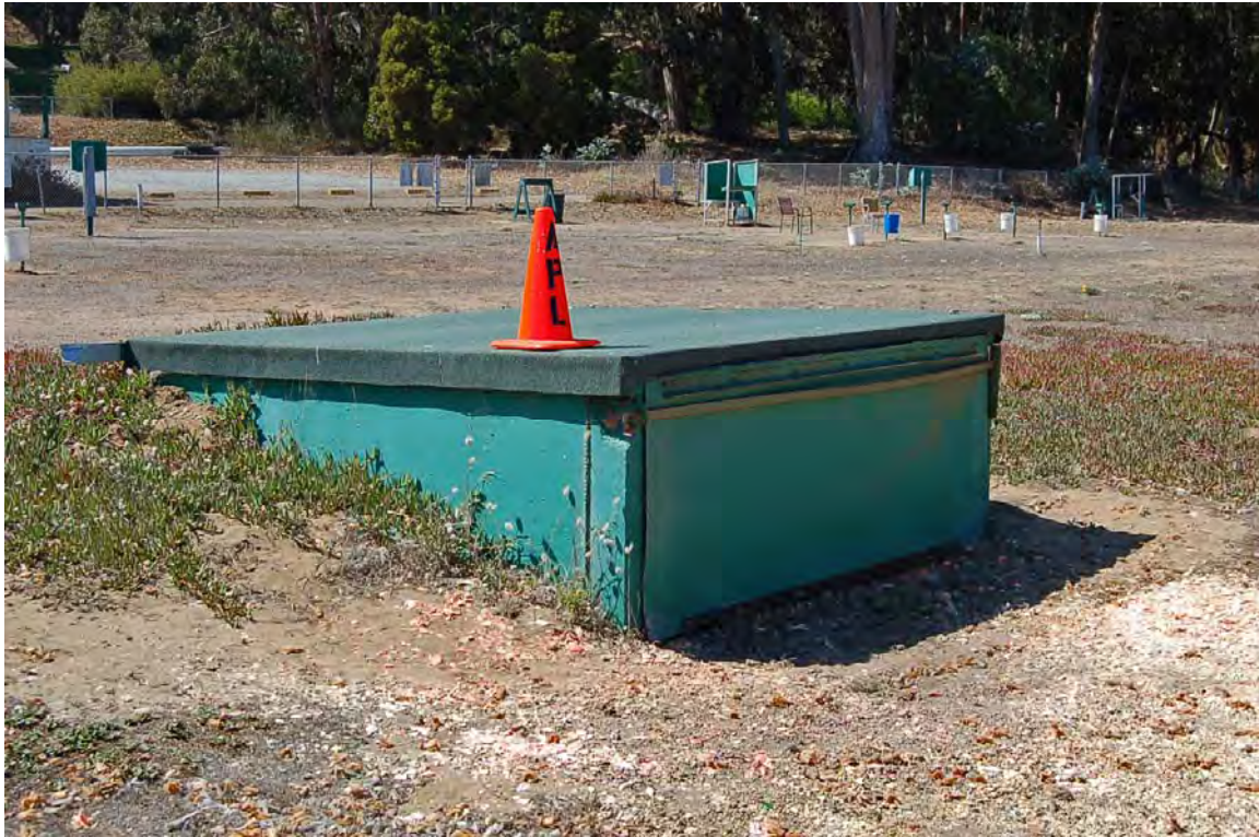
Photo 30. Trap house located at the north end of Field 3 (typical to Fields 1, 2, and 3); view to W (D. Bradley, September 2013).
