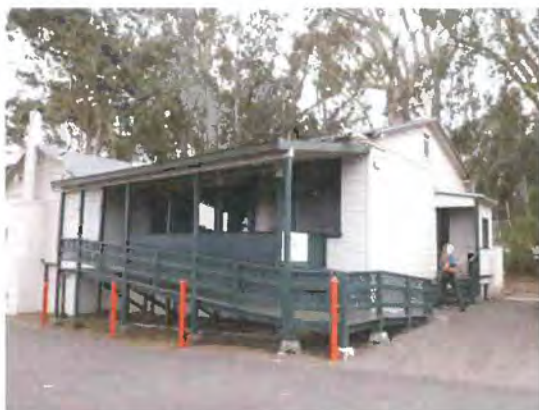
Figure 59. North façade of ell and west façade. Source: Page & Turnbull, 2013
