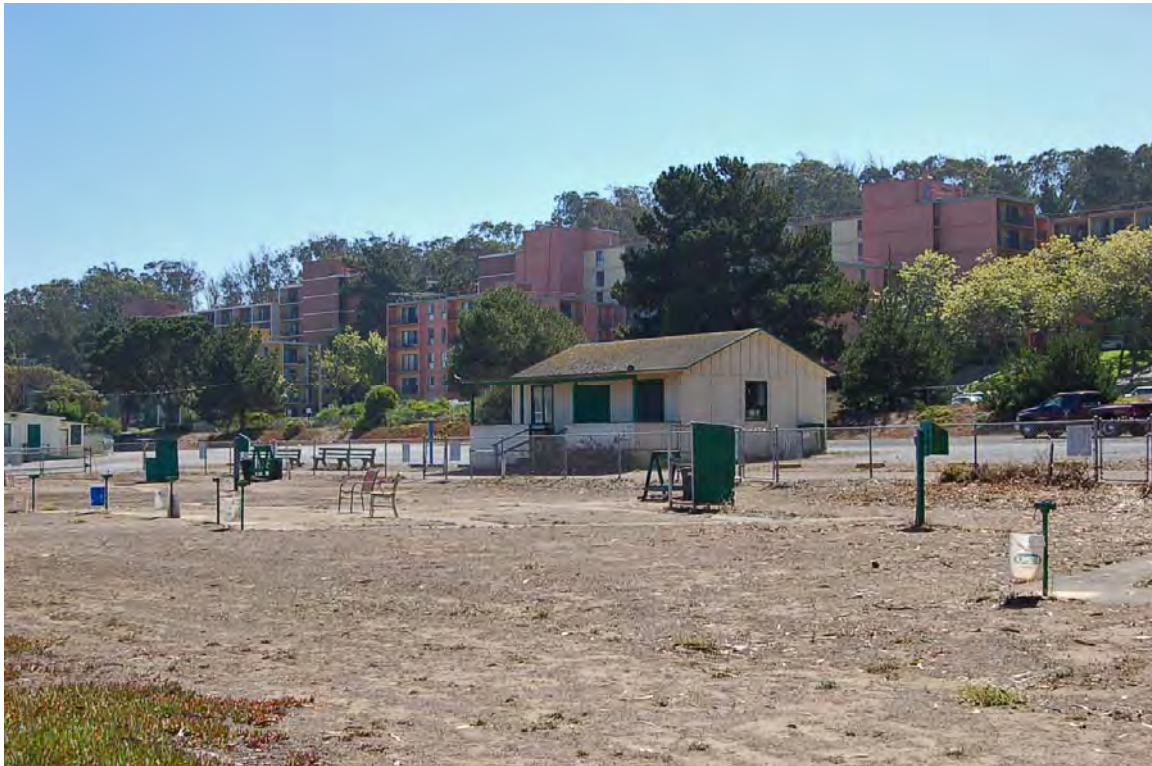
Photo 9. Trap House; view to S with trap fields in foreground (D. Bradley, September 2013).
