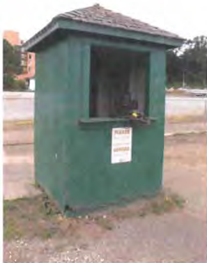
Figure 76. Hip-roofed skeet field support building. Source: Page & Turnbull, 2013
