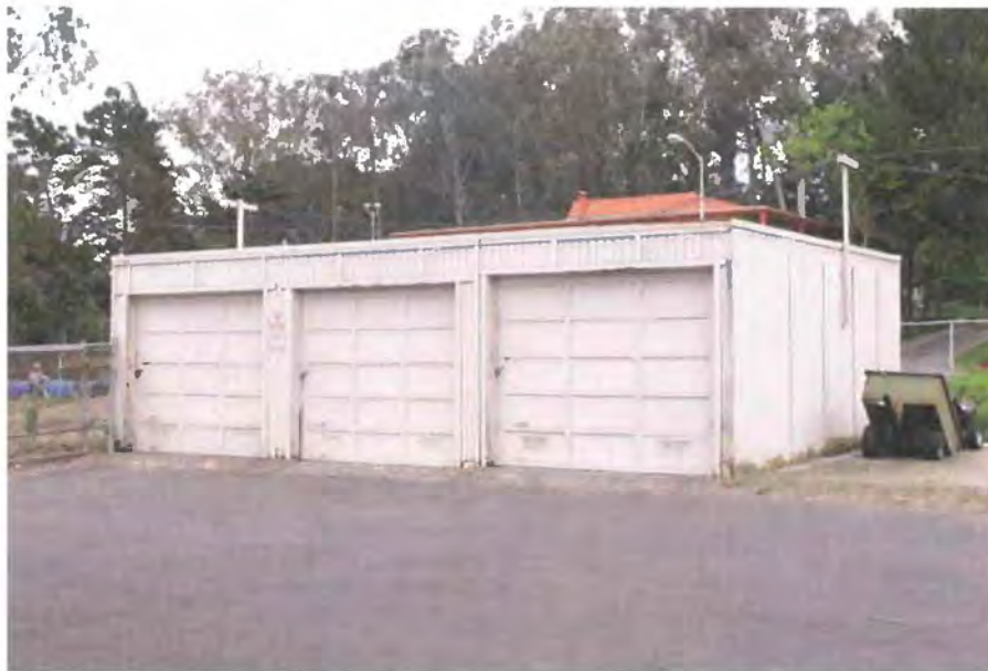
Figure 46. North façade of the Garage, viewed facing south Source: Page & Turnbull, 2013
