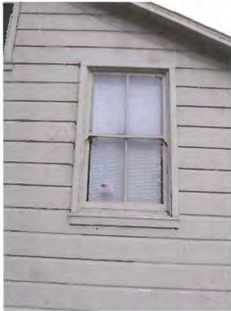
Figure 41. Detail of window on southwest façade. Source: Page & Turnbull, 2013
