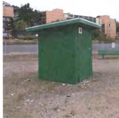
Figure 77. Shed-roofed skeet field support building. Source: Page & Turnbull, 2013
