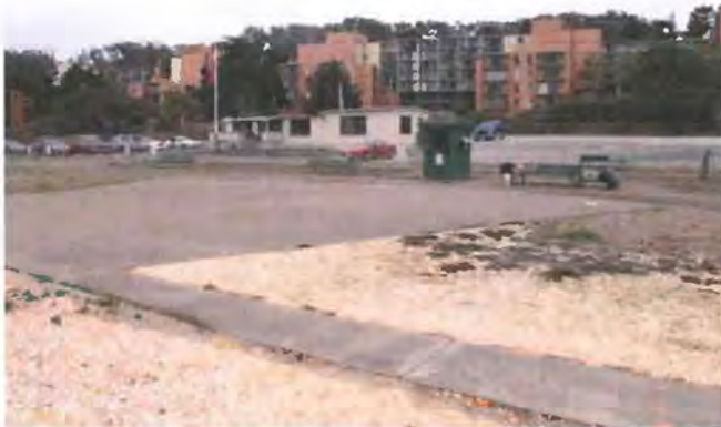
Figure 15. Concrete apron on Field 4 Source: Page & Turnbull, 2013
