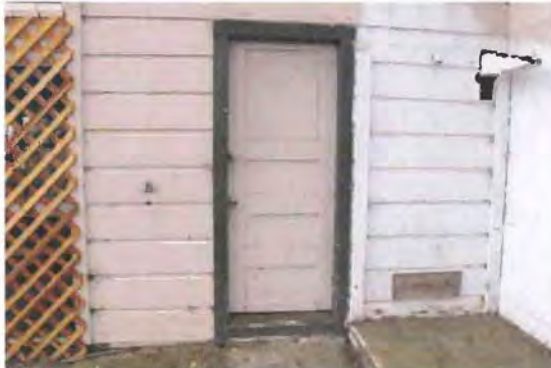
Figure 57. Detail of basement door on north façade. Source: Page & Turnbull, 2013
