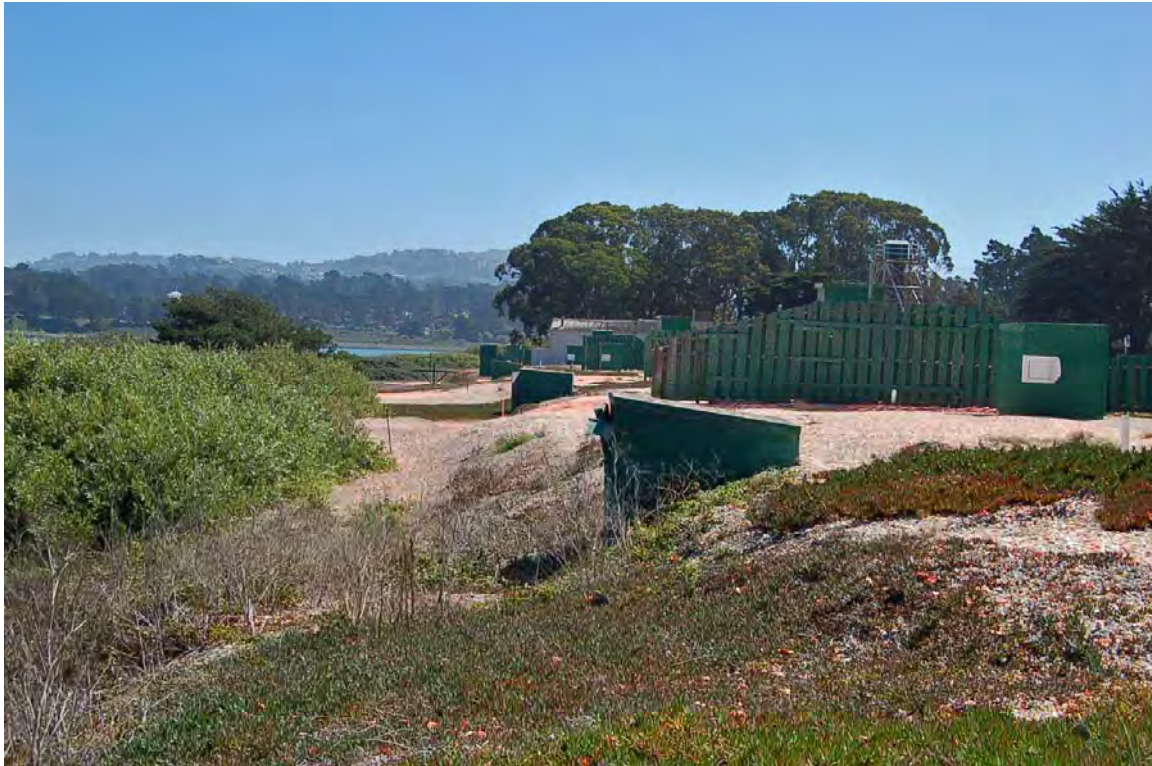
Photo 22. Skeet field complex showing topographic modifications (level fields and slope toward lake) and vegetation along shoreline; view to SE (Fields 4 to 7) (D. Bradley, September 2013).
