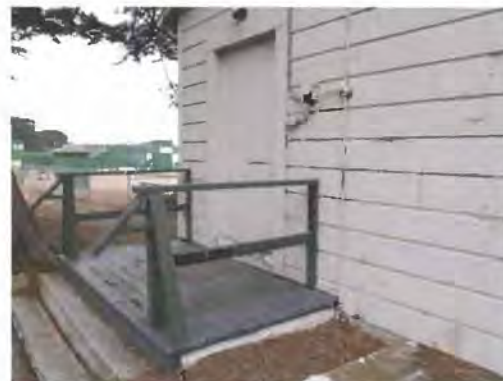
Figure 40. Detail of landing on southeast façade. Source: Page & Turnbull, 2013
