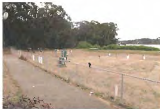
Figure 11. Primary concrete sidewalk alongside the trap fields. Source: Page & Turnbull, 2013
