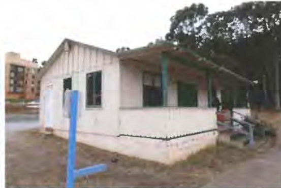
Figure 29. Southeast and northeast facades, viewed facing west.
