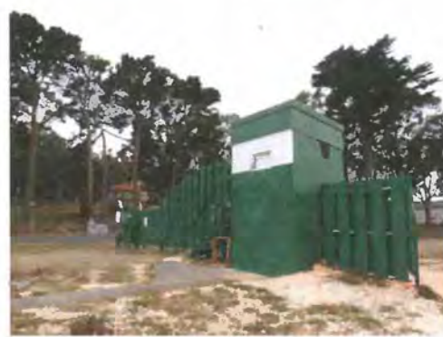
Figure 73. Combined high house/low house. between Fields 8 and 9 Source: Page & Turnbull, 2013
