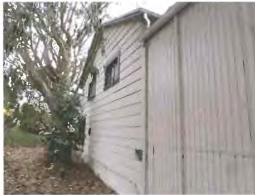
Figure 63. East end of south façade. Source: Page & Turnbull, 2013
