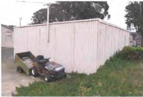
Figure 47. West facade Source: Page & Turnbull, 2013
