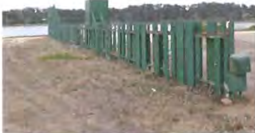
Figure 83. Protection fence between skeet fields. Source: Page & Turnbull, 2013
