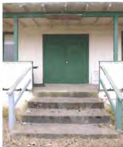
Figure 30. Paired, primary door on northeast façade within porch.
