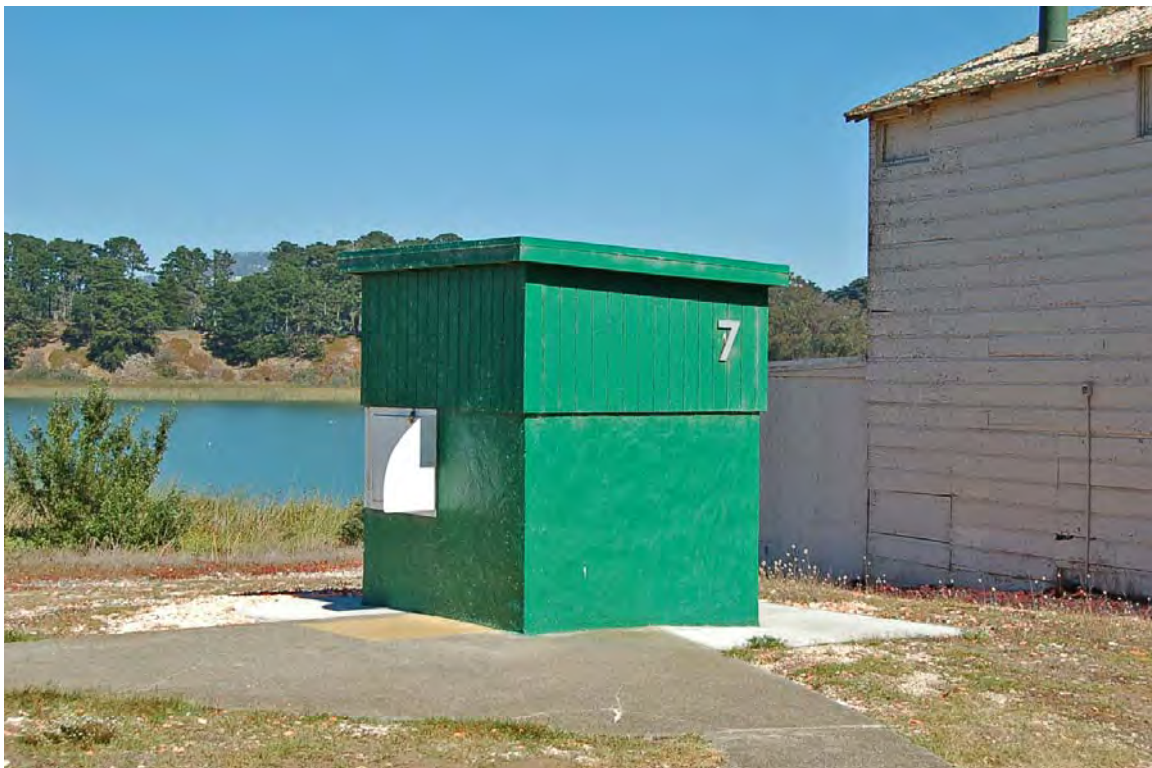
Photo 13. Low House on Field 7 (typical example of feature found on Fields 4 to 7 and 9); view to NE (D. Bradley, September 2013).
