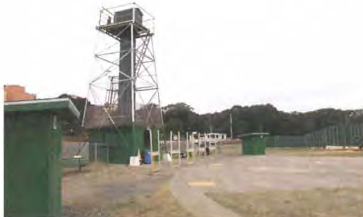
Figure 81. Duck tower and Field 6, viewed facing north. Source: Page & Turnbull, 2013
