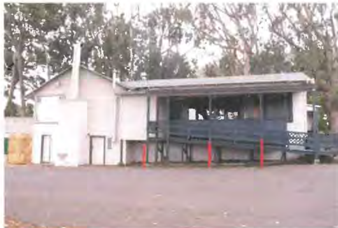
Figure 55. East and north facades of the Club House, viewed facing southwest. Source: Page & Turnbull, 2013
