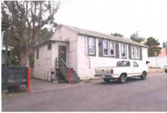
Figure 50. East and north facades, viewed facing southwest Source: Page & Turnbull, 2013
