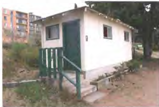
Figure 37. Southeast and northeast facades Source: Page & Turnbull, 2013
