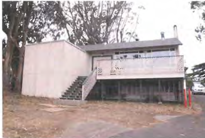
Figure 64. East façade. Source: Page & Turnbull, 2013
