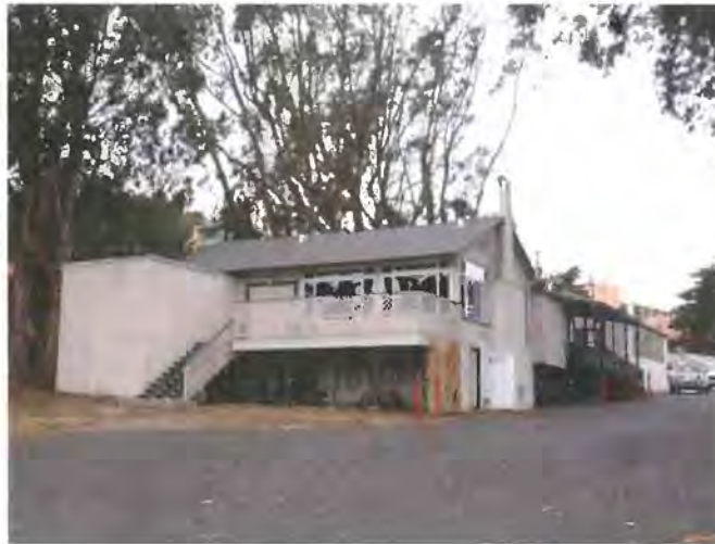
Figure 54. East and north facades of the Club House, viewed facing southwest. Source: Page & Turnbull, 2013
