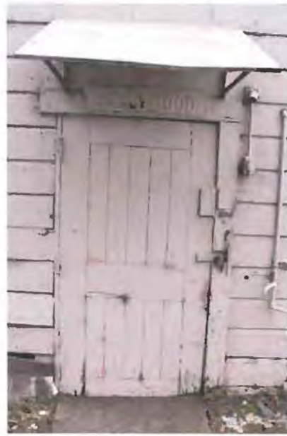
Figure 42. Basement door on southeast façade. Source: Page & Turnbull, 2013
