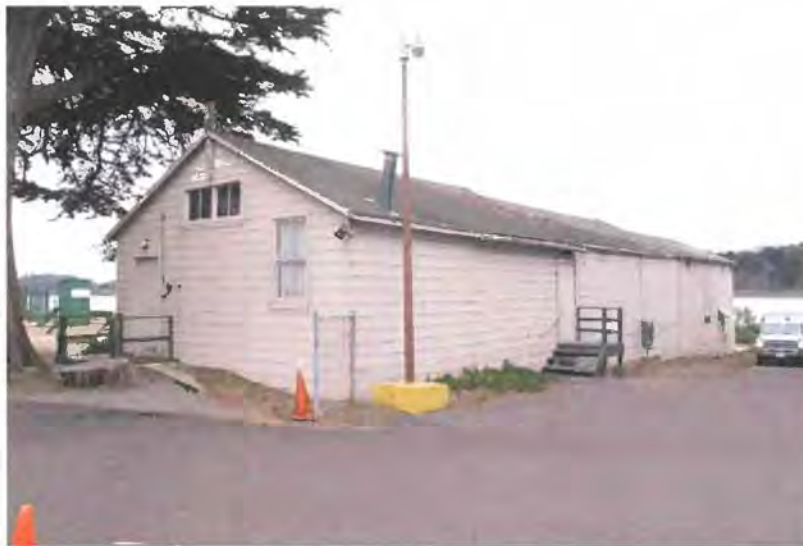
Figure 38. Southwest and southeast facades, viewed facing north
