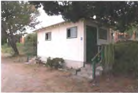
Figure 36. Northeast and northwest facades Source: Page & Turnbull, 2013
