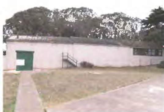
Figure 44. Northwest façade. Source: Page & Turnbull, 2013
