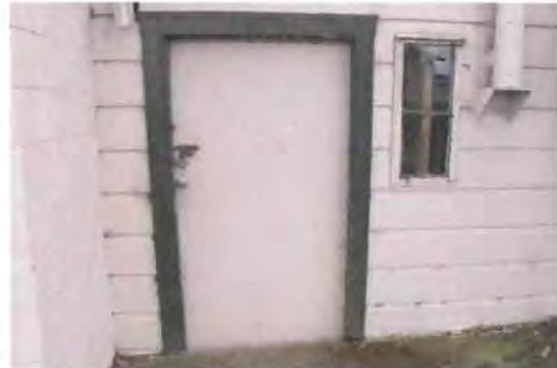
Figure 58. Detail of basement door on north façade. Source: Page & Turnbull, 2013
