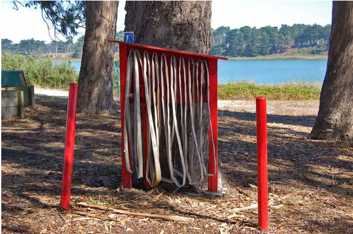
Photo 42. Fire hose (D. Bradley, September 2013).
