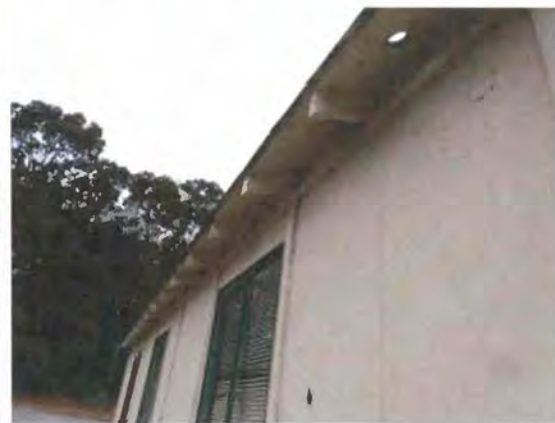
Figure 34. Rafter tails under eaves on southwest façade. Source: Page & Turnbull, 2013
