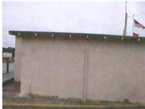
Figure 26. West end of southwest façade. Source: Page & Turnbull, 2013
