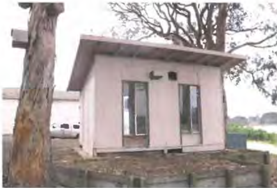
Figure 65. South façade of shed Source: Page & Turnbull, 2013
