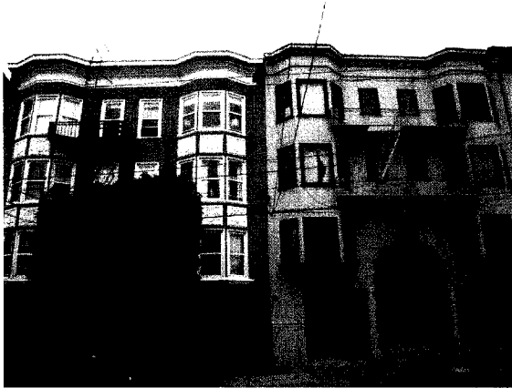
1. NEIGHBORING PROPERTY (VIEW FROM FILBERT ST.)
