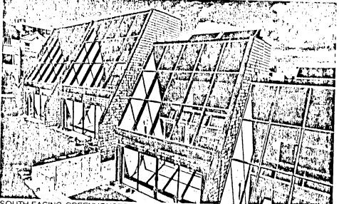
SOUTH-FACING GREENHOUSES on Sunhouse townhouses in San Francisco present 406 sq. ft. of glazing at an angle perpendicular to the noon sun on December 31. The pussive system is expected to provide over 70 percent of the heating load for the \$200,000 units.
