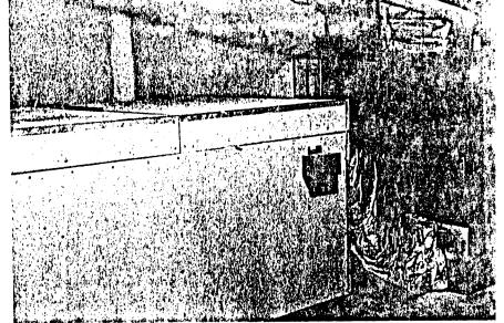
EUTECTIC SALT STORAGE is housed in a container fabricated of wallboard phase-change medium can store a relatively great amount of heat in a small vo
