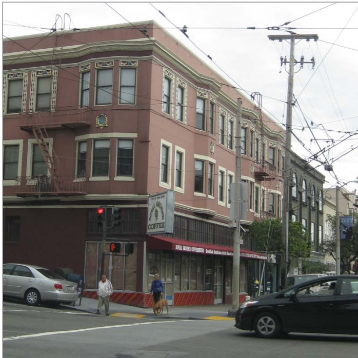
Figure VIII-12. The Former Royal Ground Coffee Shop at Fillmore and California Streets, Site of a Future Rag & Bone Clothing Boutique (a Formula Retail Use Approved by the Commission in February 2014)
