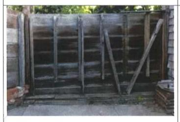
North exterior wall. Note the level floor line at the bottom of the original framing studs.
