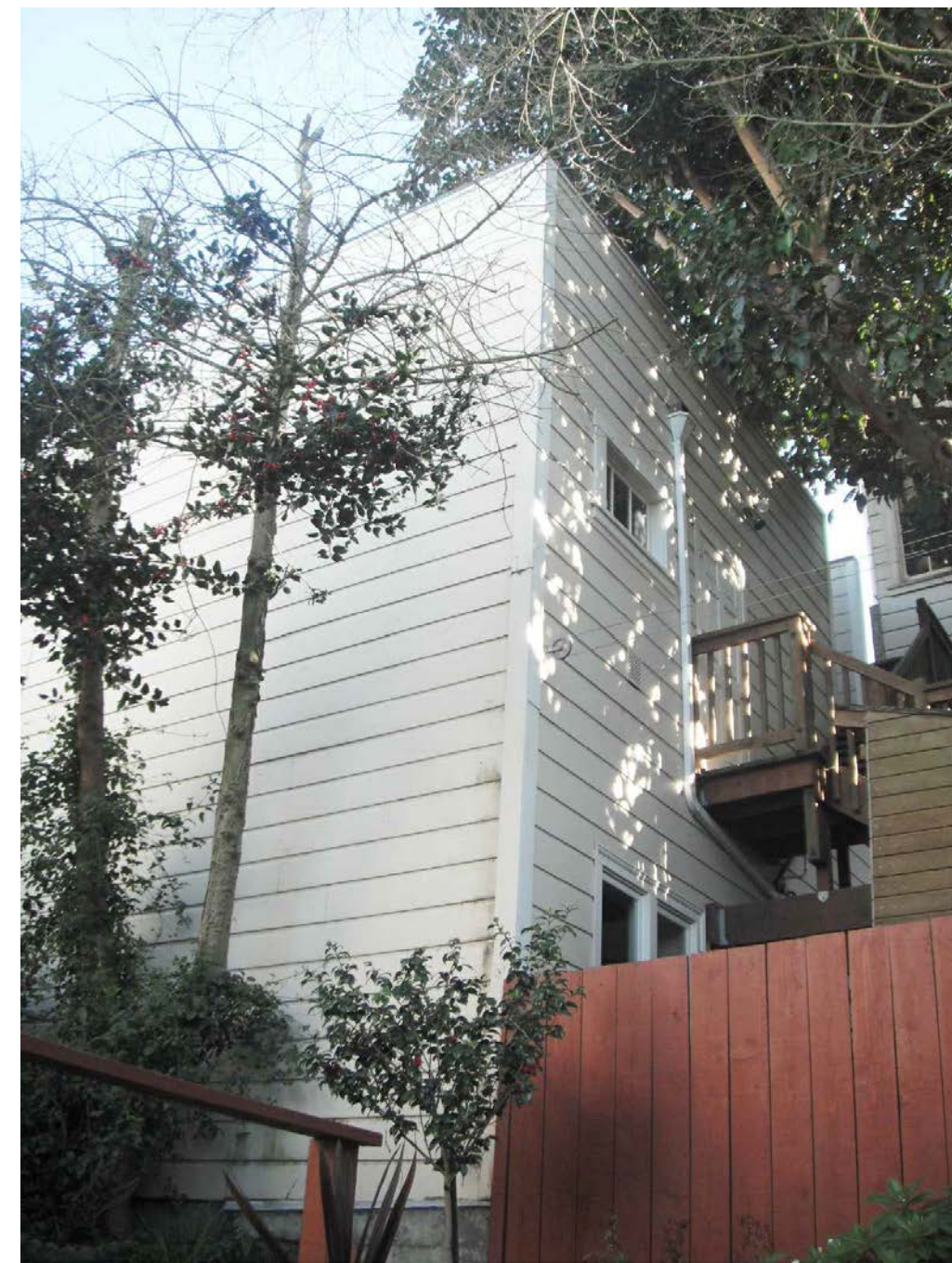
3 VIEW FROM REAR YARD
