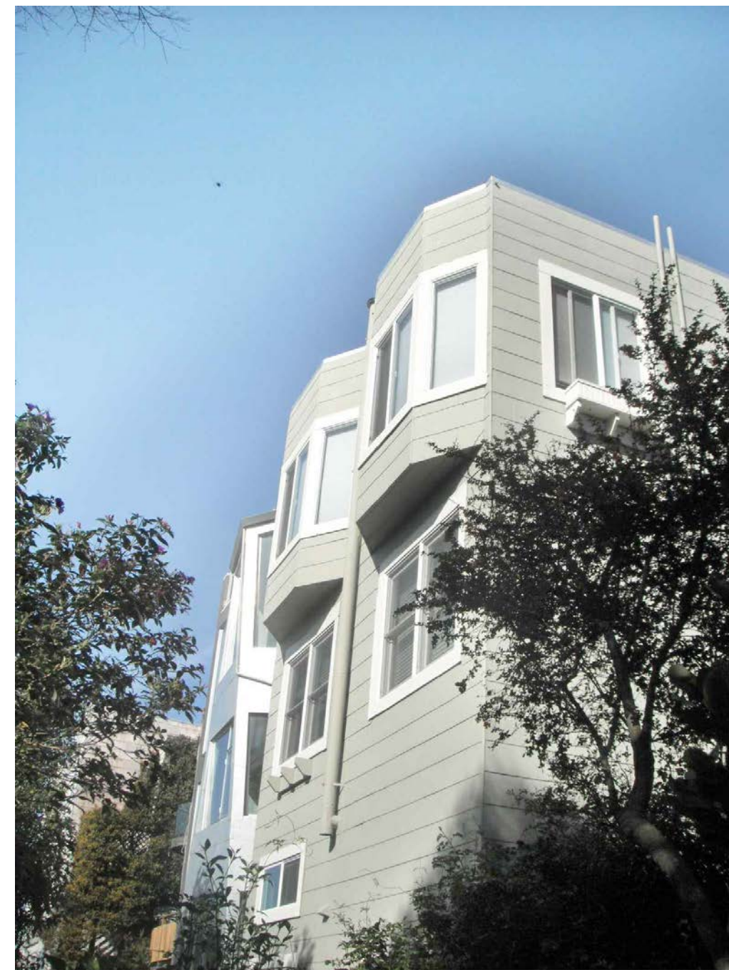
2 VIEW FROM REAR YARD
