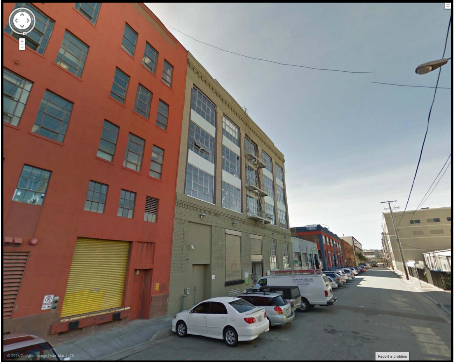
410 Townsend Street, View along Bluxome Street
