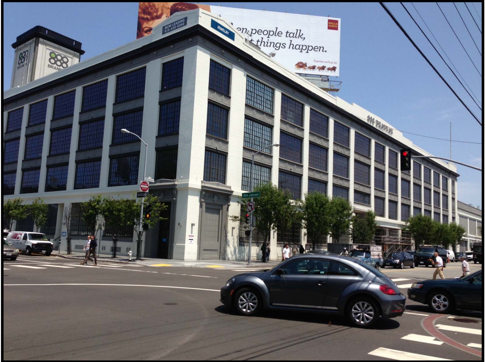
870 Brannan Street, Brannan Street Facade
