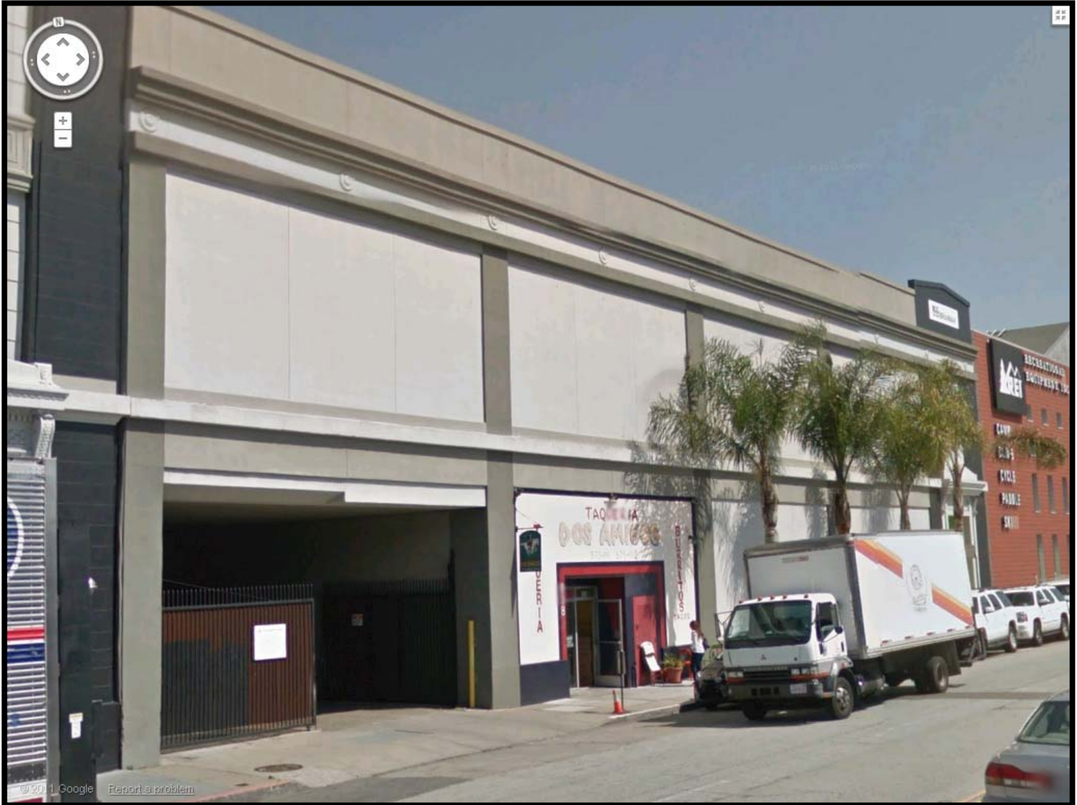
850 Brannan Street, Brannan Street Façade
