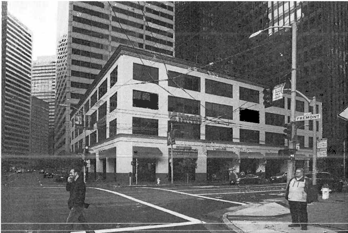
Previous Condition (Building on site has been demolished)
