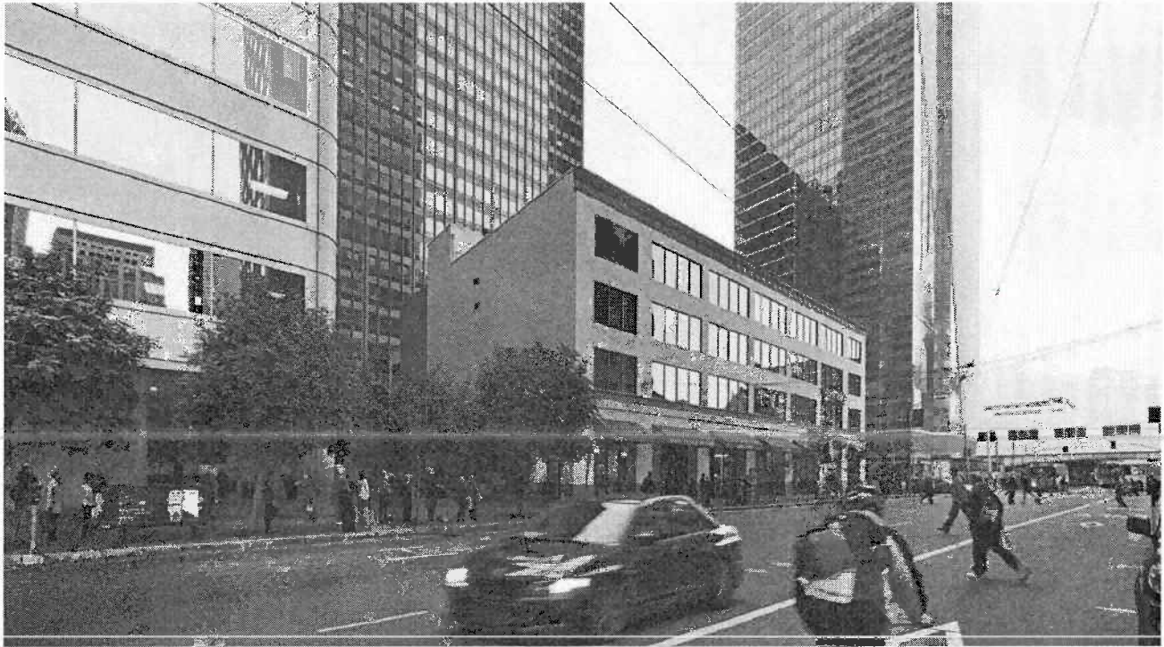
Previous Condition (Building on site has been demolished)
