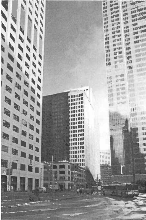
Previous Condition (Building on site has been demolished)
