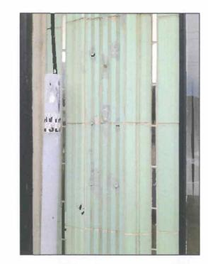
PHOTO A: DAMAGED TILE DETAIL AT LEFT PILASTER
