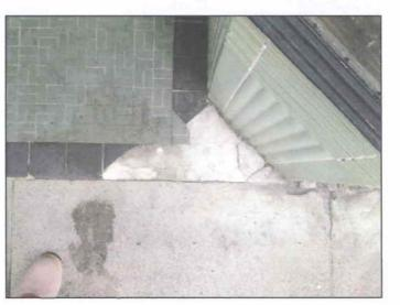
PHOTO C: DAMAGED TILE DETAIL AT HISTORICAL ENTRY
