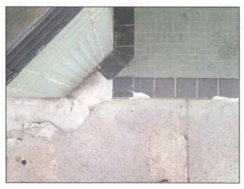
PHOTO B: DAMAGED TILE DETAIL AT HISTORICAL ENTRY
