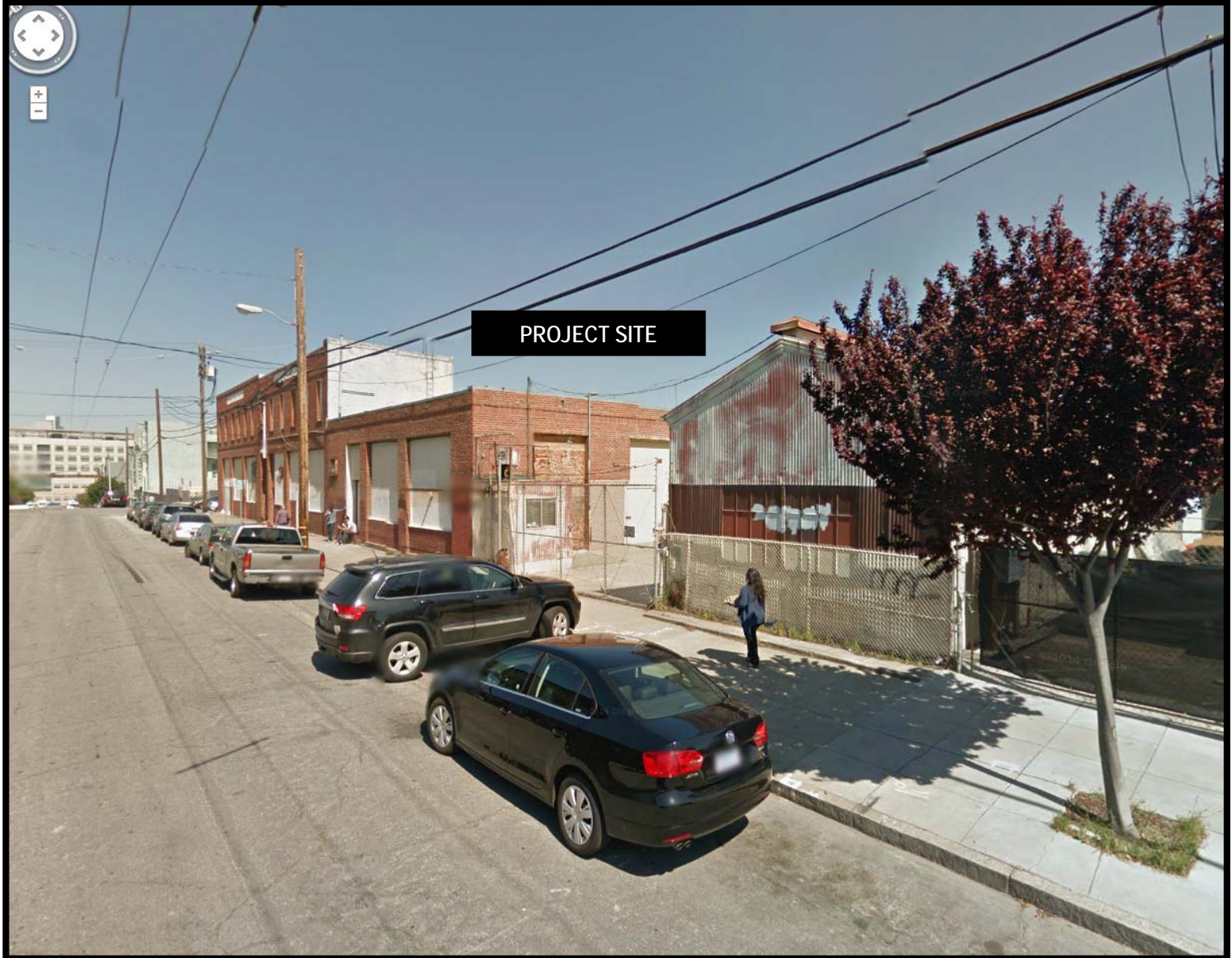
815-825 Tennessee Street, View along Tennessee Street
