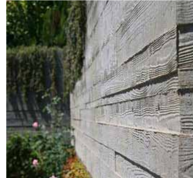
Board Formed Concrete
