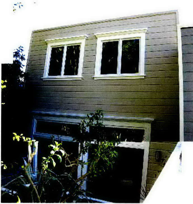
REAR OF ADJACENT PROPERTY 16 VICKSBURG 3627/006
