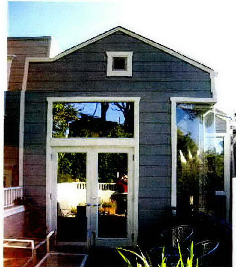
REAR OF SUBJECT PROPERTY 18 VICKSBURG 3627/007
