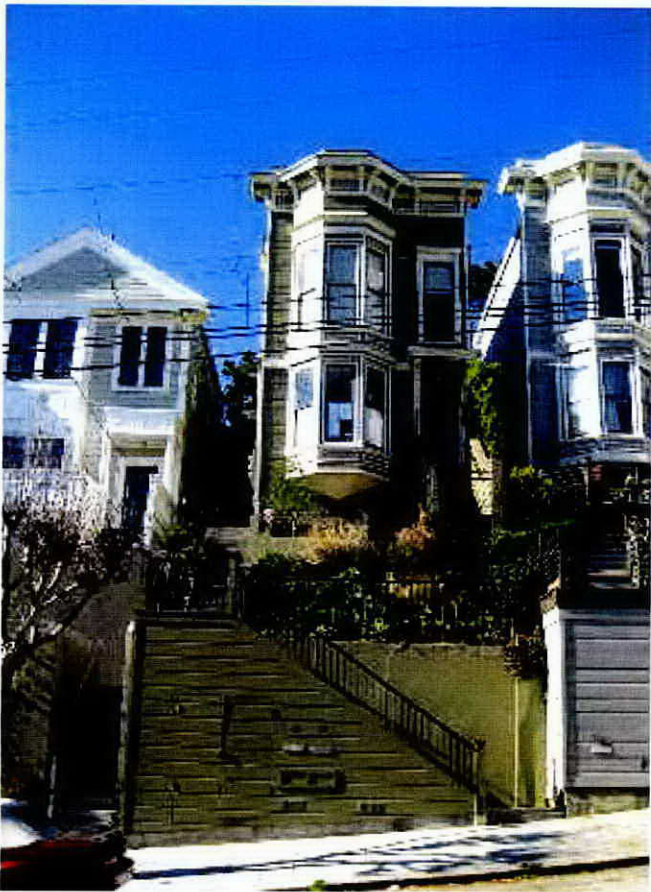
FRONT OF ADJACENT PROPERTY 20-22 VICKSBURG ST. 3627/008
