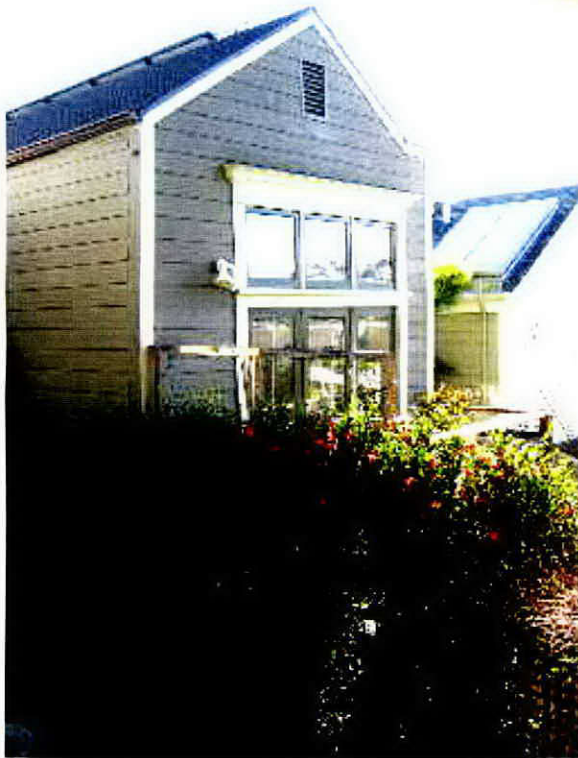
REAR OF ADJACENT PROPERTY 20-22 VICKSBURG 3627/008
