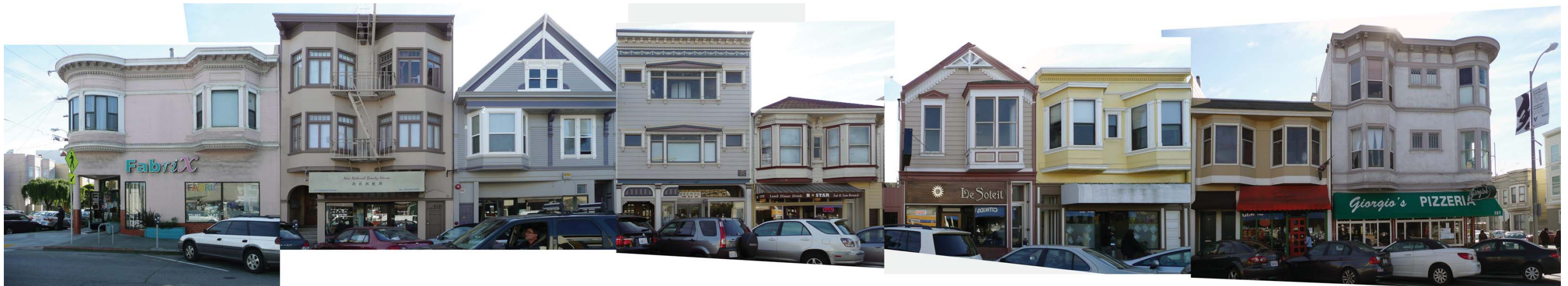
BLOCK PHOTO OF CLEMENT STREET (LOOKING SOUTH)
