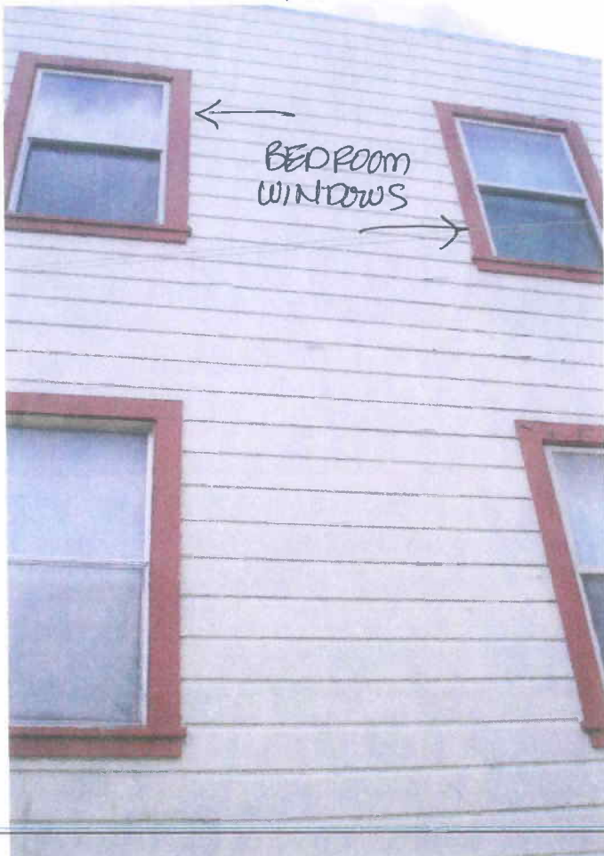
REAR OF LOT 16C STRUCTURE
