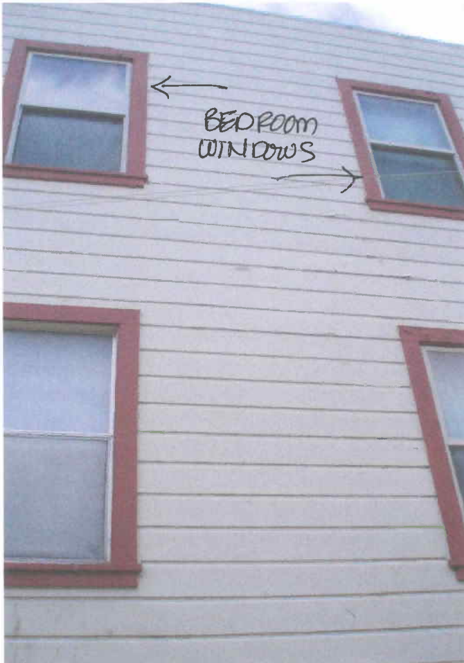
REAR OF LOT 16C STRUCTURE
