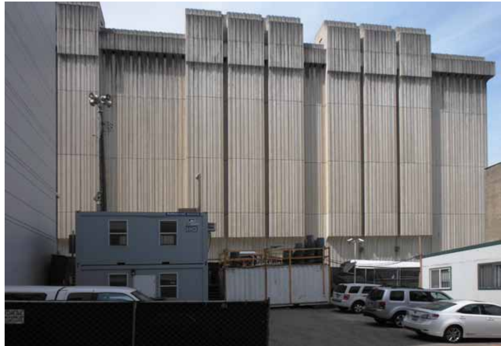
View 8: Photograph of Site looking towards PG&E Substation from Zeno Place
