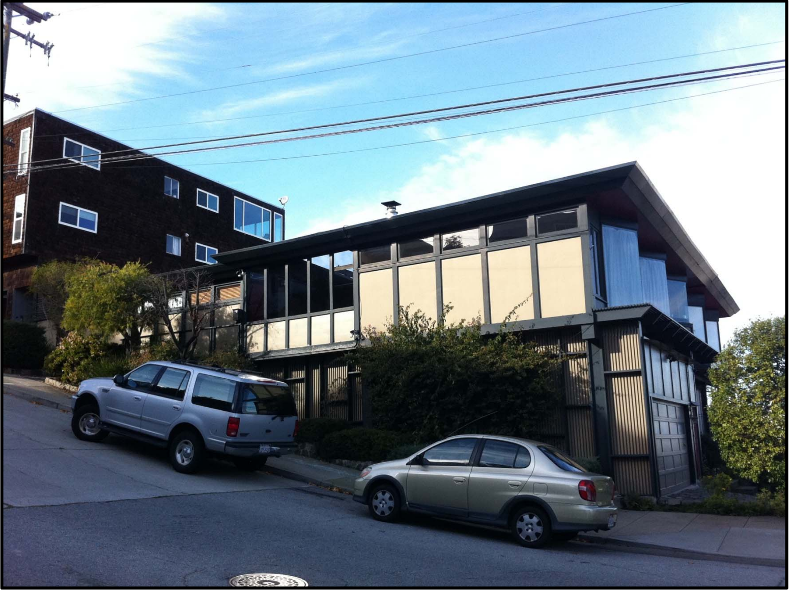
2000 20 th Street, View of 20 th Street
