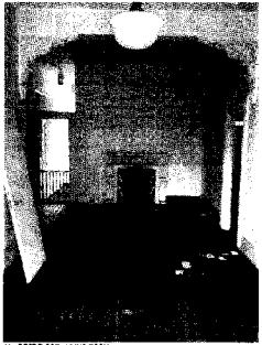
07 - FIRST FLOOR - LIVING ROOM
