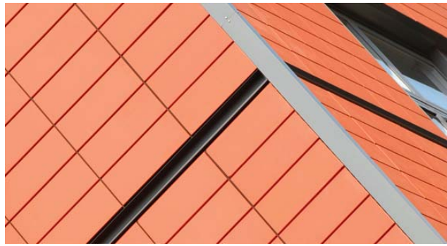
DETAIL SHOWING TILES & TRIM
