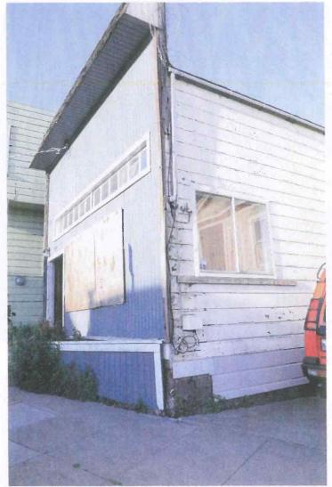
N/E corner of 882 Carolina St., depicting deteriorating condition, foundation and temporary vinyl siding covering up fire damage.
