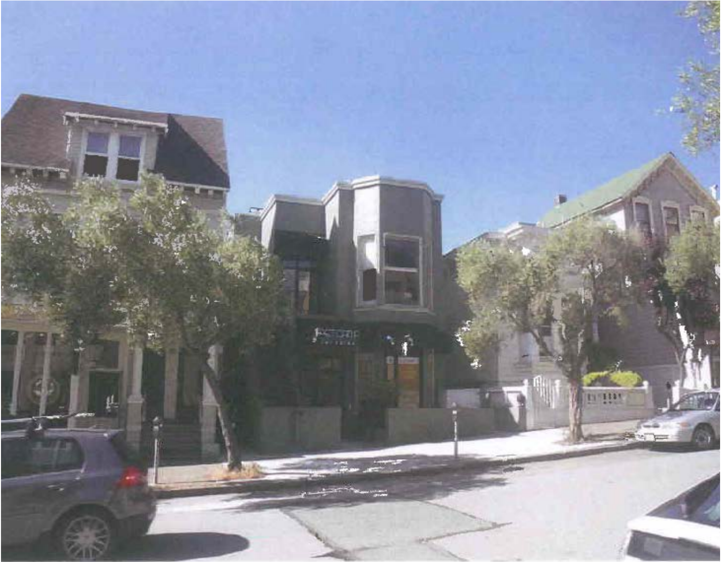
Subject Property center, taken from Sacramento St. towards Lyon St.
