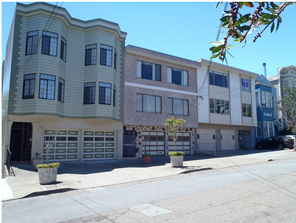
This block of Hill St is at the very edge of the Liberty-Hill Historic District's southeast boundary, and reflects a typical San Francisco neighborhood-with a mix of both historic and contemporary buildings. Of the 17 buildings on the south (Project) side of Hill St, less than half are listed in the California Historical Resources Inventory and/or City-adopted surveys, according to the Planning Department. More than a third of the buildings on Hill St contain multiple units and at least five buildings contain five units or more.
