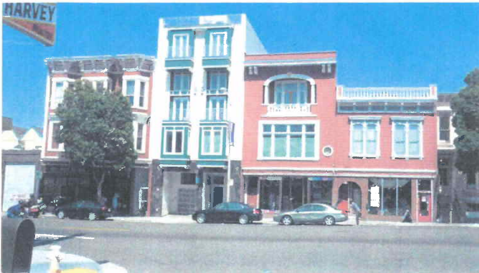
Victorian buildings directly across the street from 1050 Valencia
