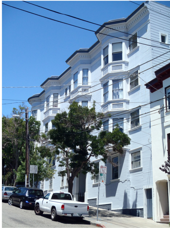
The four story, historical building at 98 Hill and Guerrero streets contains 13 units, about the same density -and on an almost identical sized lot - as the Project.
