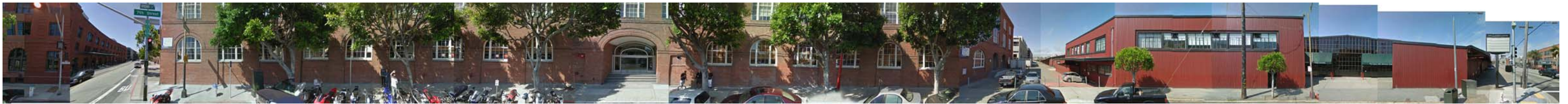
Seventh Street - East Facing
