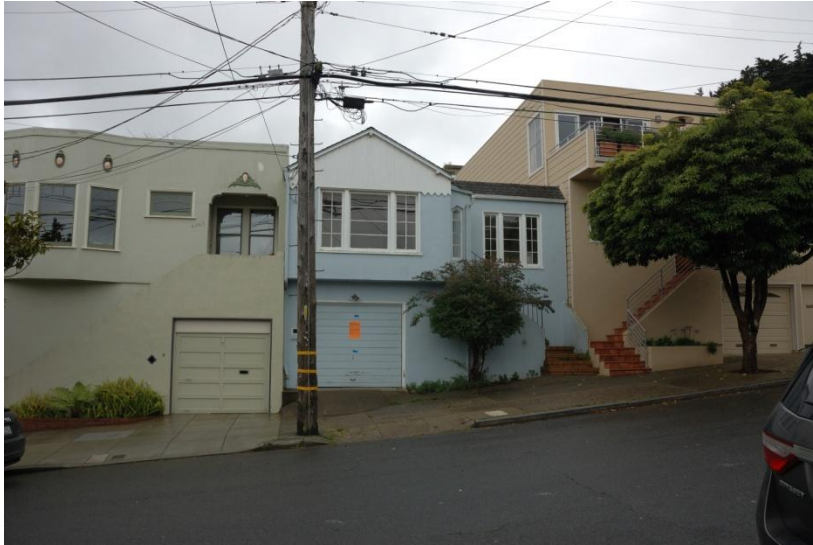
DR Requester on right, currently projects above. Proposed design creates more consistency.
