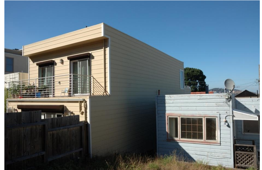
4371 projects 24' 6" from rear of 4365 main building and 10' 5" from rear addition.
