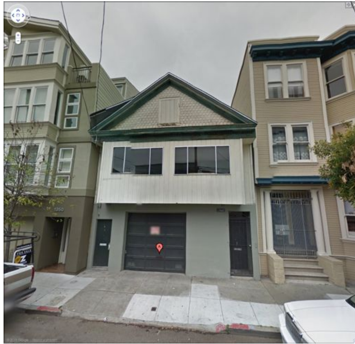
LOOKING NORTHWEST: FROM NATOMA STREET: PROJECT SITE: BUILDING TO BE DEMOLISHED.
