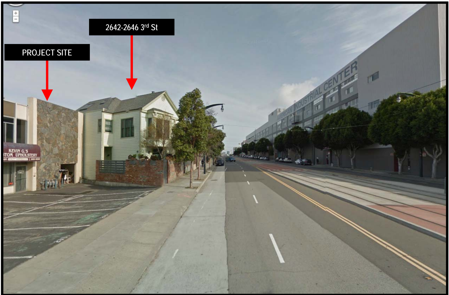
1201-1225 Tennessee Street, View along 3 rd Street and Adjacent Property
