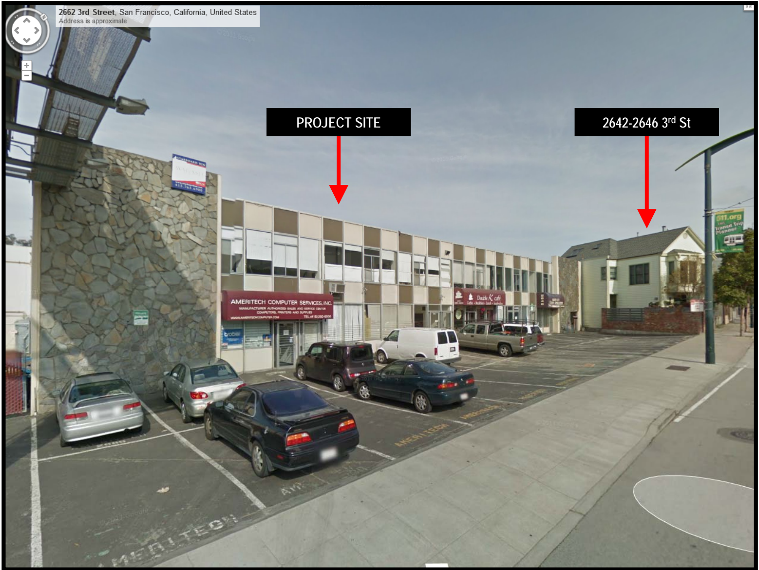
1201-1225 Tennessee Street, View along 3 rd Street
