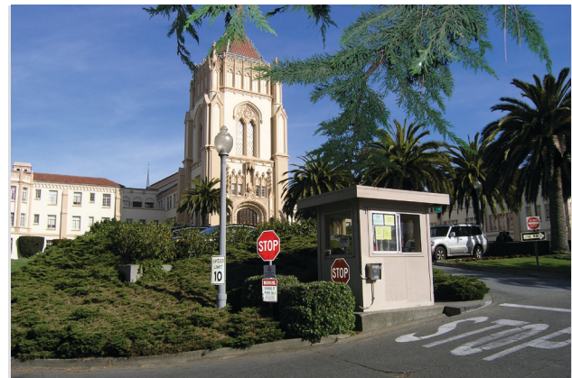
Entry point lacks identity
