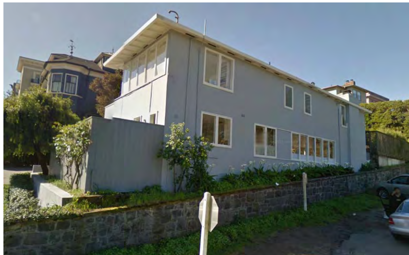
Figure 6. North façade, March 2011. Source: Google Maps ©2012 Google.
