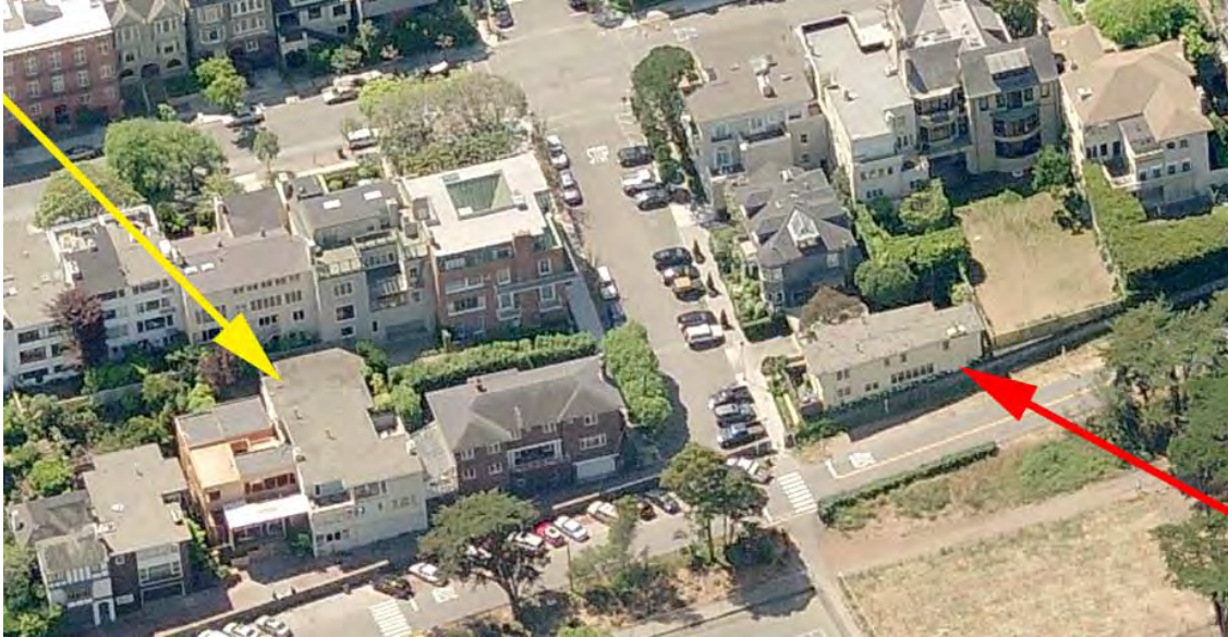
Figure 9. Aerial view looking south, with red arrow pointing to One Spruce Street and yellow arrow pointing to 16 Spruce Street.
