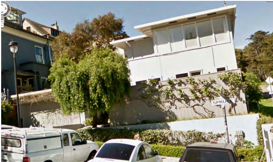
Figure 4. Primary (east) façade, April 2011. Source: Google Maps ©2012 Google.
