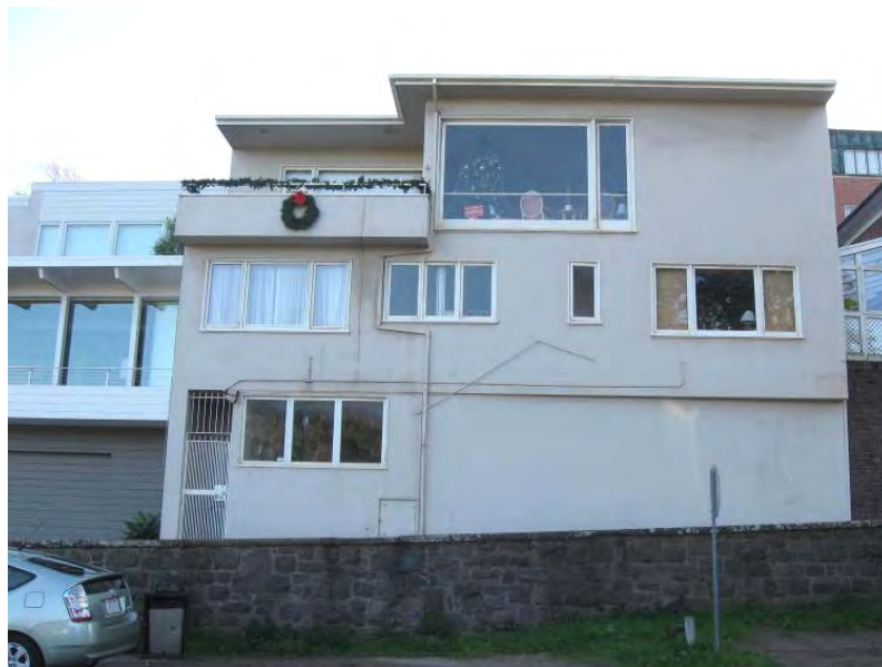
Figure 10. 16 Spruce Street, north (rear) façade on Pacific Avenue. Designed in 1946 by Ward and Bolles, Architects.
