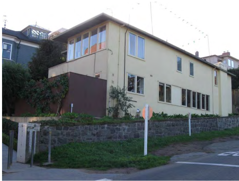
Figure 5. North façade, looking southwest. Source: Page & Turnbull, December 2009.
