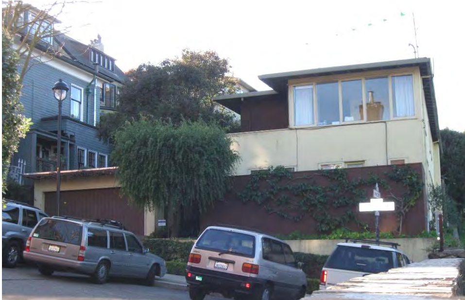
Figure 3. Primary (east) façade. Source: Page & Turnbull, December 2009.
