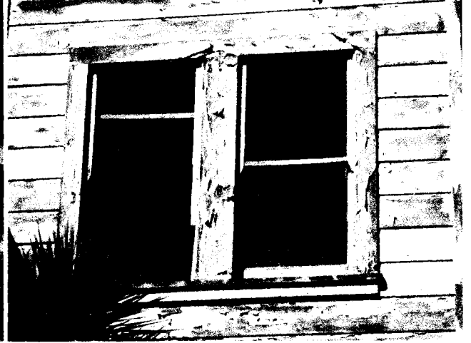
Photo 20: Damaged & Deteriorated Rear Windows
