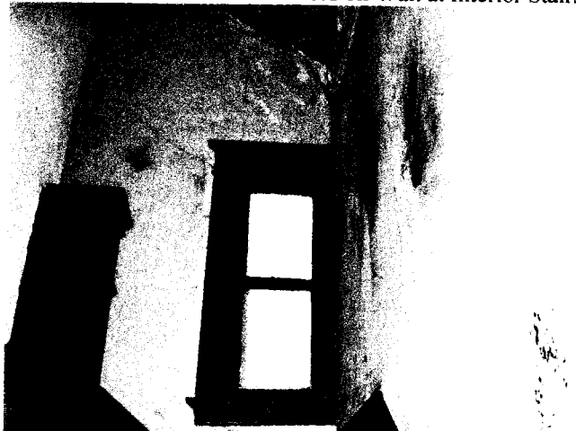
Photo 41: Wall & Ceiling Damage at Interior Stairs
