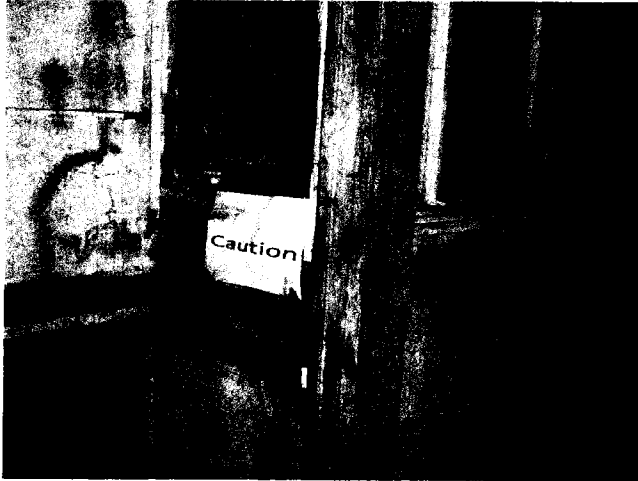
Photo 55: Wood Decay and Damage at Kitchen Window
