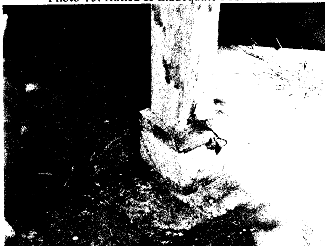
Photo 17: Inadequate Post Base Connection
