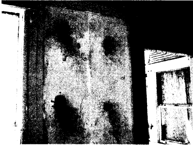
Photo 73: Damages on Rear Bedroom Wall
