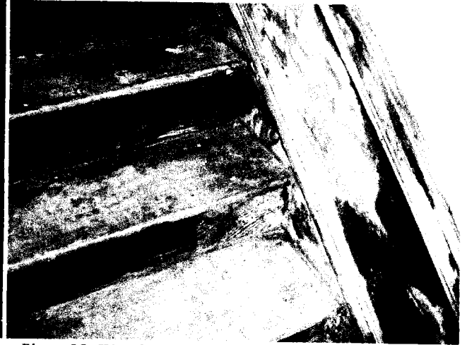
Photo 38: Wood Decay at Interior Stairs
