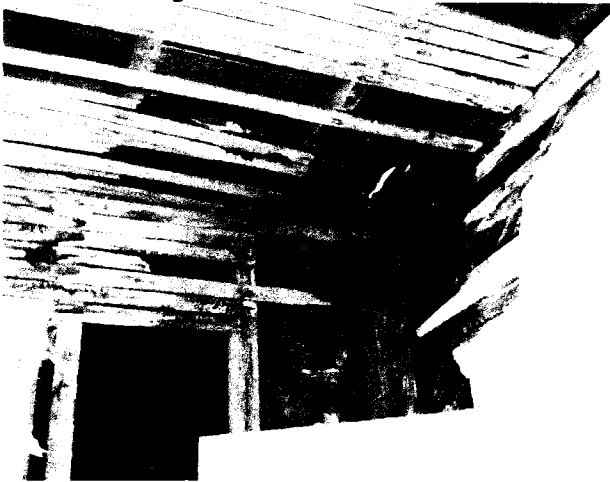
Photo 75: Severe Framing Deterioration at Sunroom
