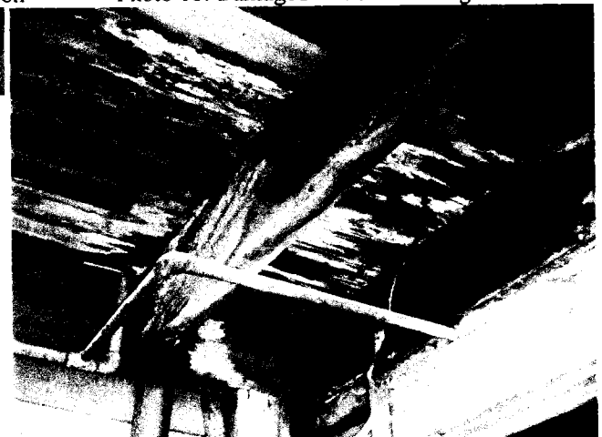
Photo 18: Rotted Laundry Room Floor Framing
