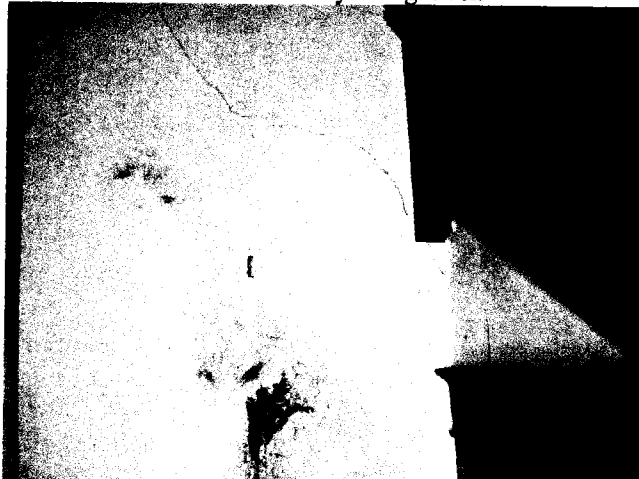
Photo 35: Settlement Crack & Possible Mold on The Wall at Foyer
