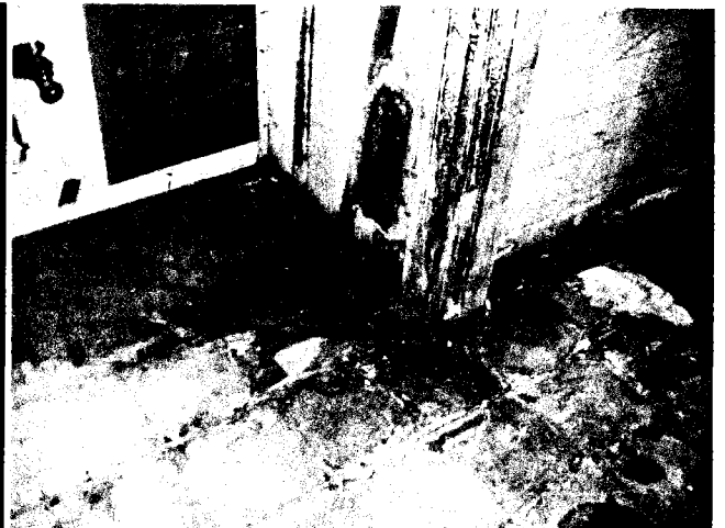
Photo 56: Wood Decay and Damage on Kitchen Floor2.
