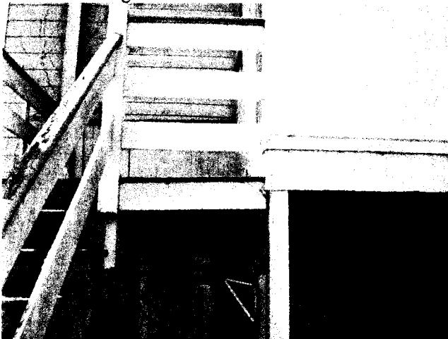
Photo 81: Questionable Framing at Rear Porch
