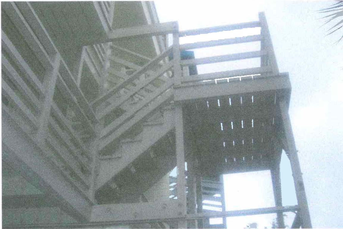
REAR VIEW TO WEST
