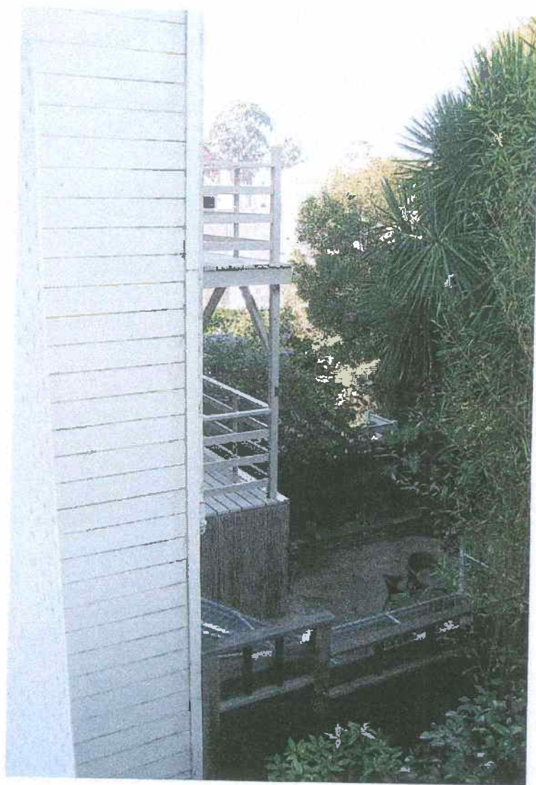
VIEW TO WEST AT REAR OF BUILDING
