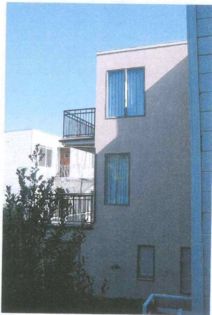
VIEW TO EAST AT REAR OF BUILDING
