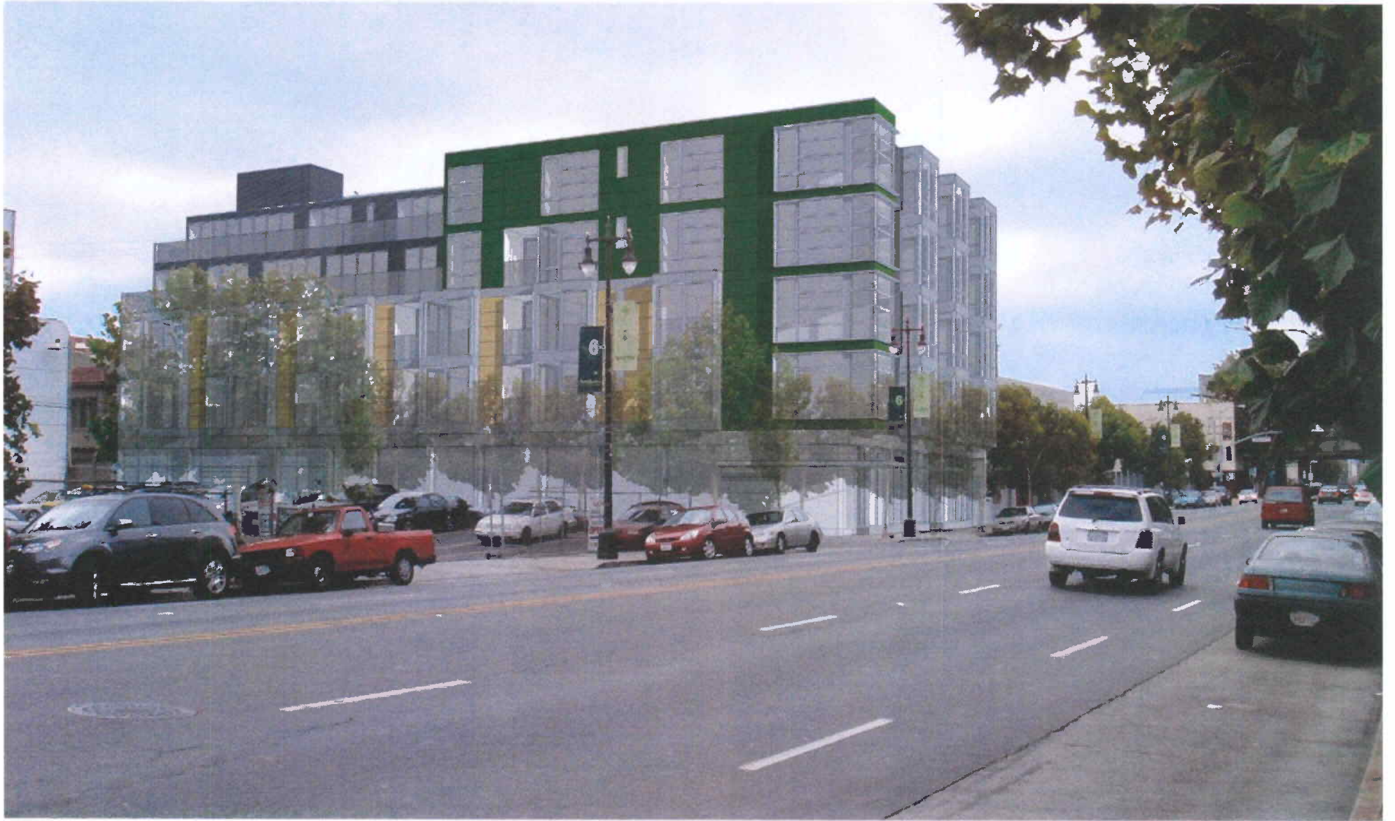
View from 6th Street, Looking South Towards 345 6th Street
