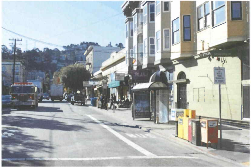
View South on Cole Street at Subject Property
