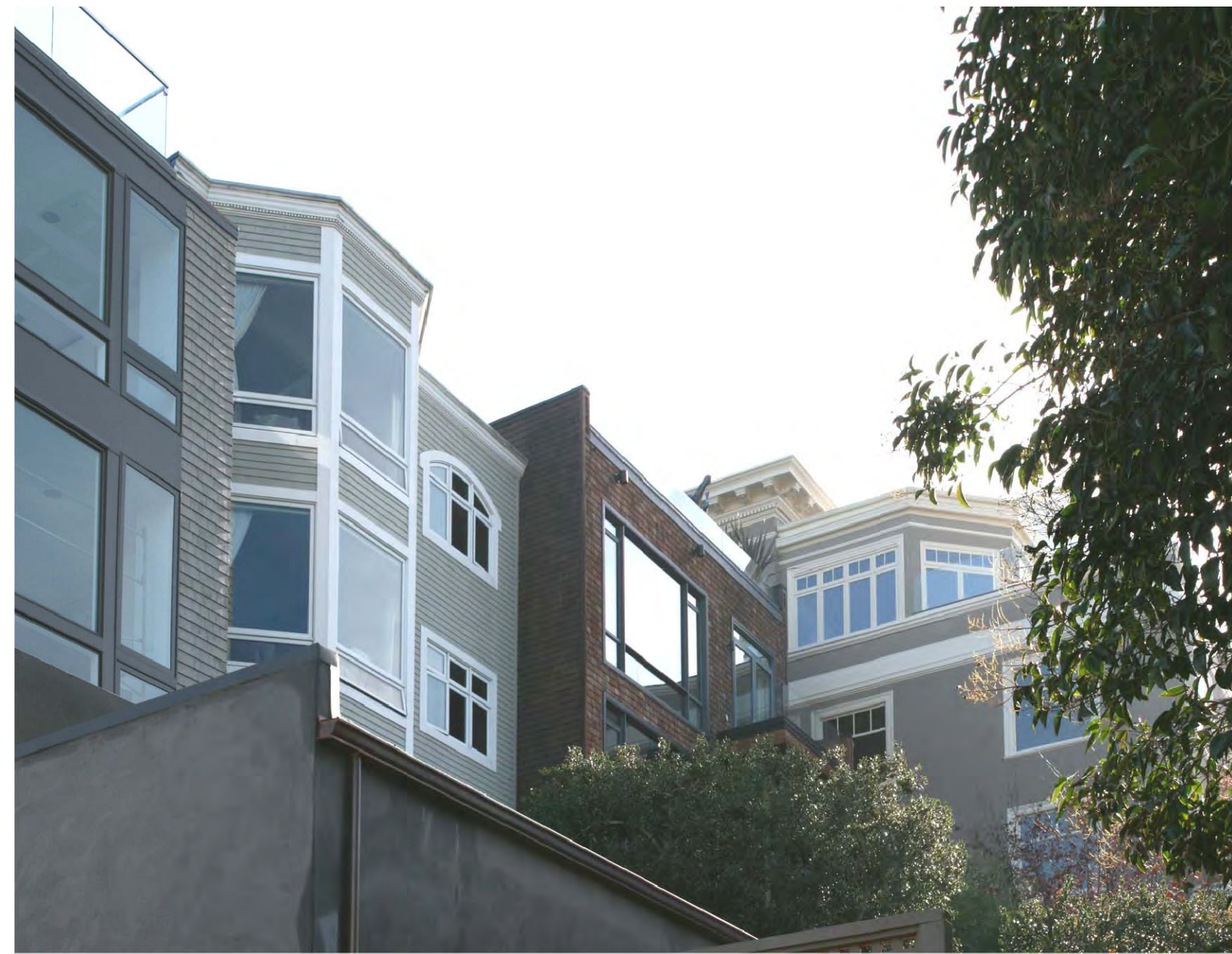
2705 & 2707 Larkin Street - Rear Facades 3 N/A A2.00
