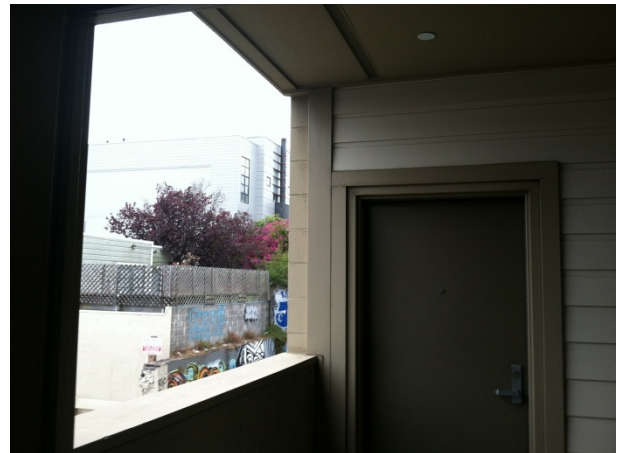
Looking SW, #105 2 nd floor door (views/ trees) [The windows to right are not shown]
