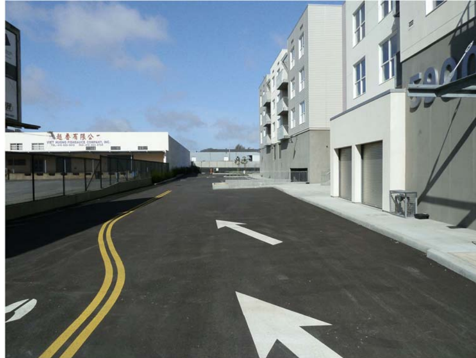
5) VIEW: BUILDING 2 AT PRIVATE RD. LOADING AREA
