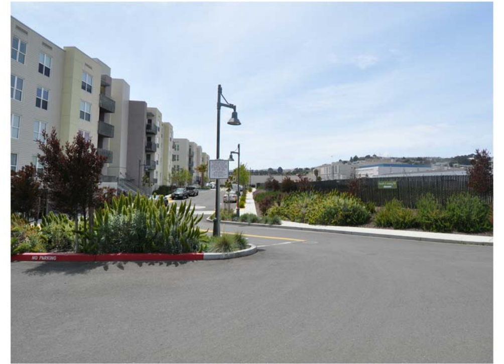
3) VIEW: PRIVATE RD. LOOKING SOUTH
