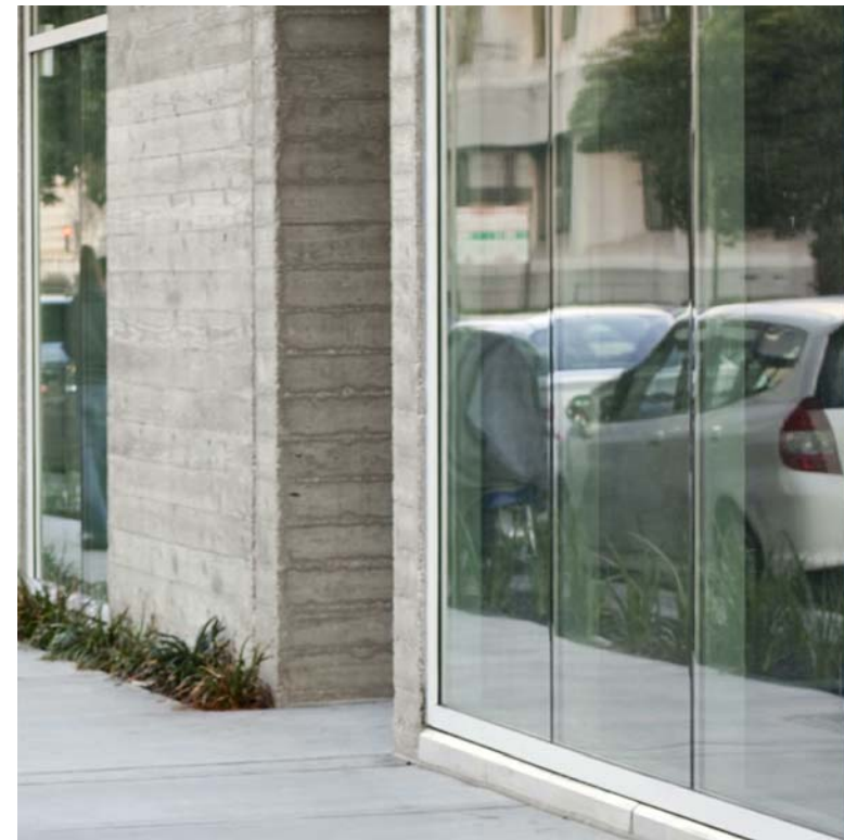
BOARD FORM CONCRETE AND STOREFRONT WINDOWS
