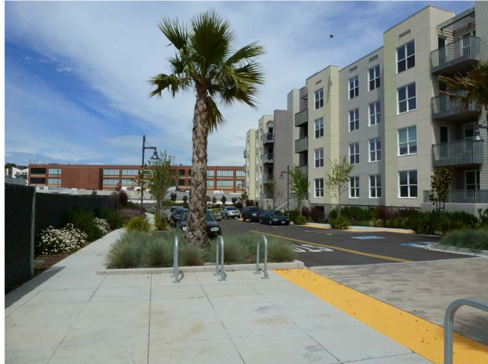
4) VIEW: BUILDING 1 FROM PRIVATE RD.
