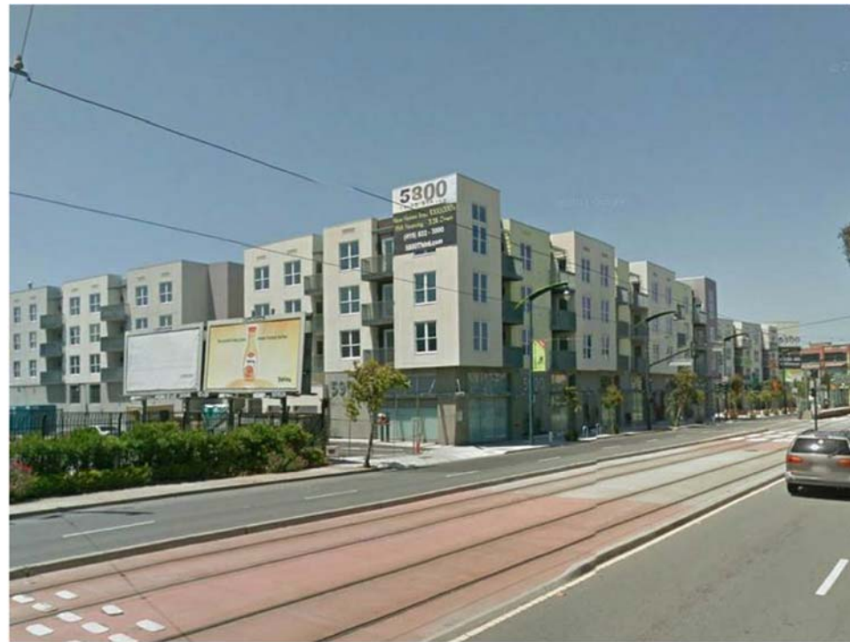
5) VIEW: BUILDINGS 1 & 2 FROM THIRD ST. LOOKING NORTH
