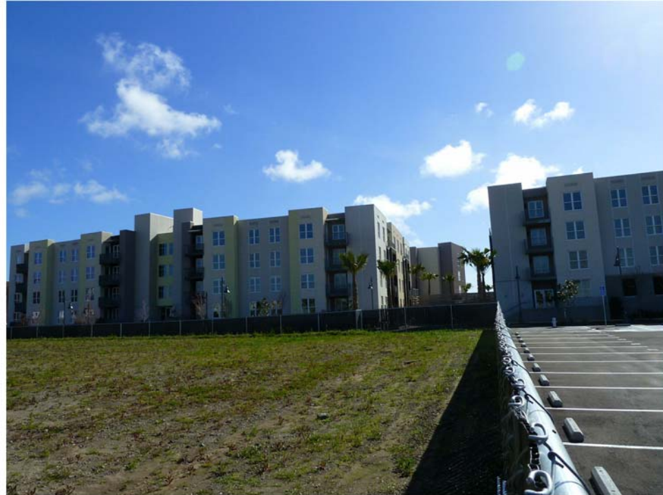
4) VIEW: LOT 42 SITE LOOKING EAST
