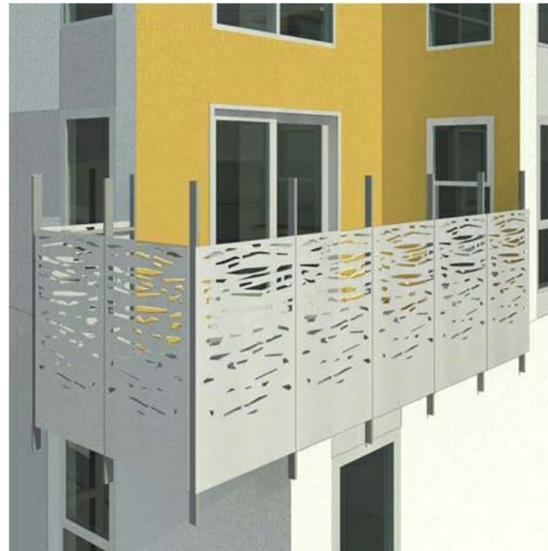
PERFORATED METEL BALCONY RAILINGS WITH AFROCENTRIC PATTERN
