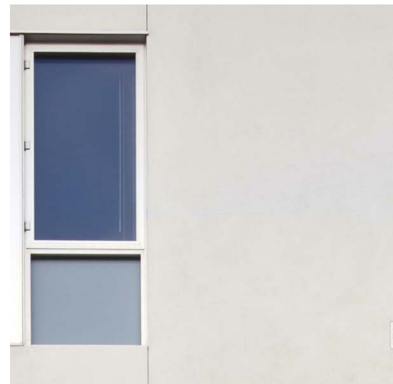
CEMENT PLASTER WITH THERMALLY BROKEN ALUMINUM WINDOWS
