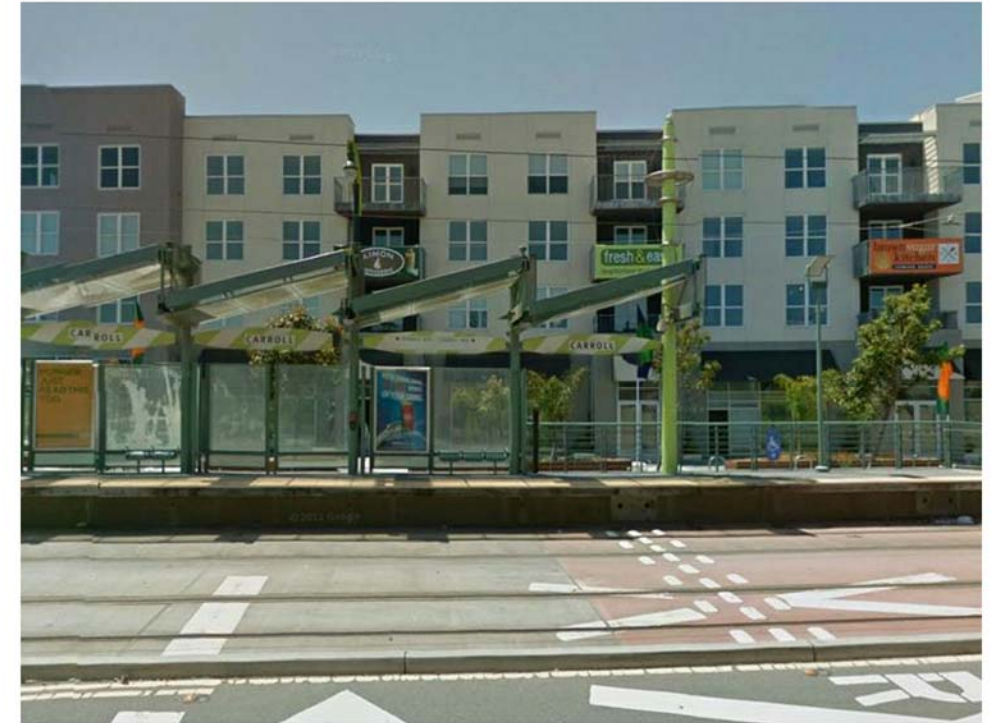
3) VIEW: BUILDING 1 FROM THIRD ST.
