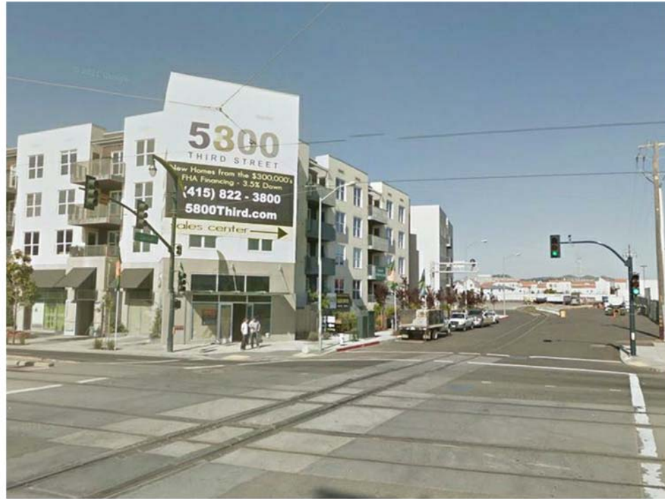
1) VIEW: BUILDING 1 FROM THIRD ST. & CARROLL AVE.
