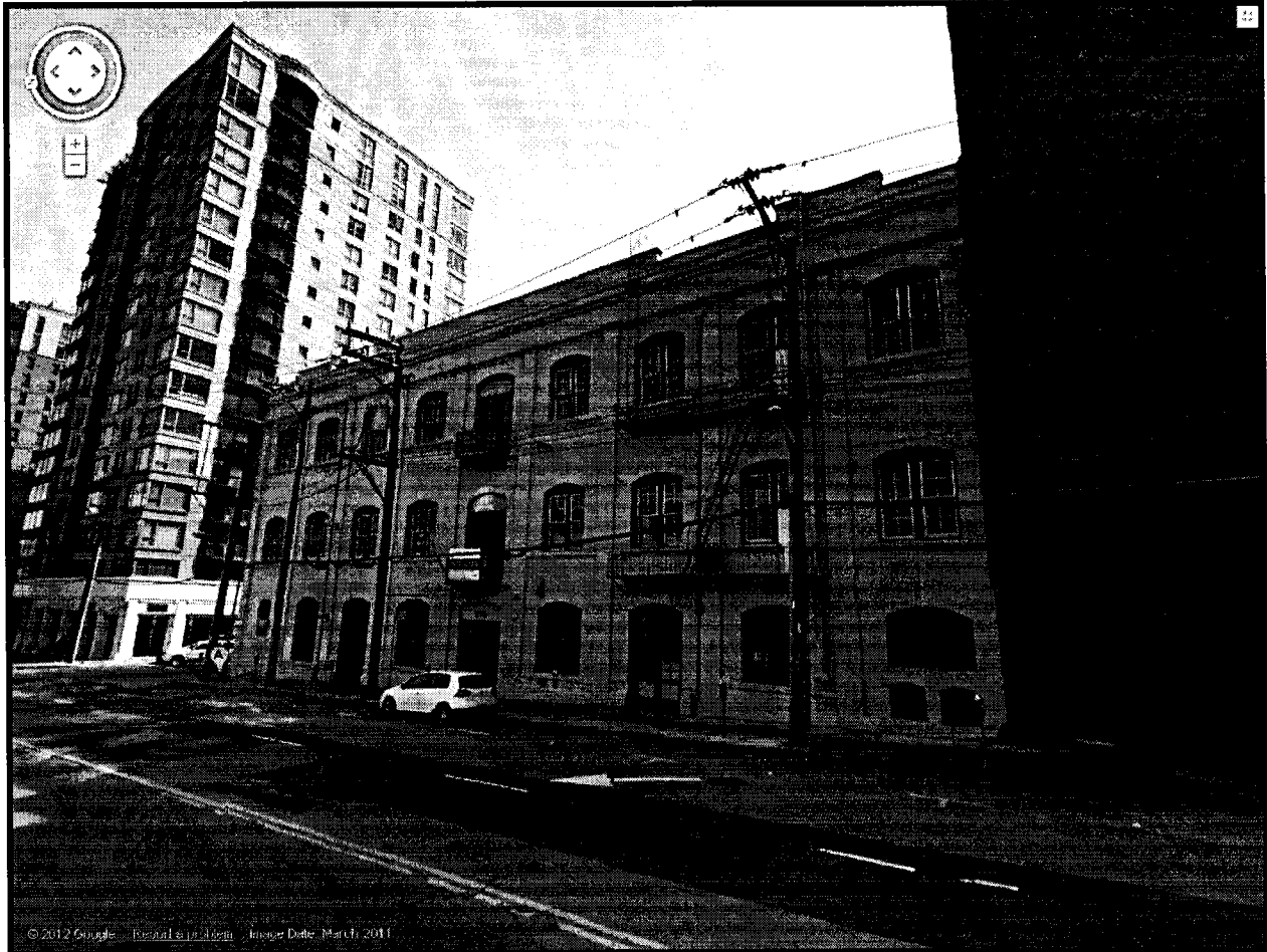
275 Brannan Street, View along Brannan Street (Source: Google Maps, Accessed May 22, 2012)
