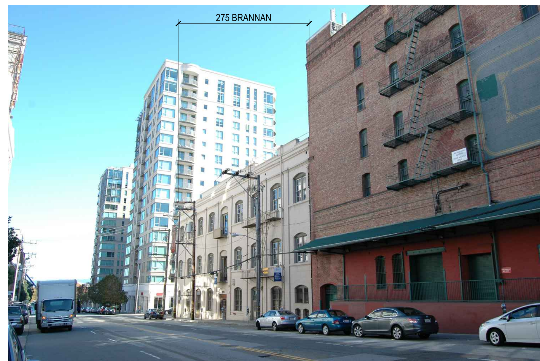
BRANNAN STREET LOOKING EAST | 3
