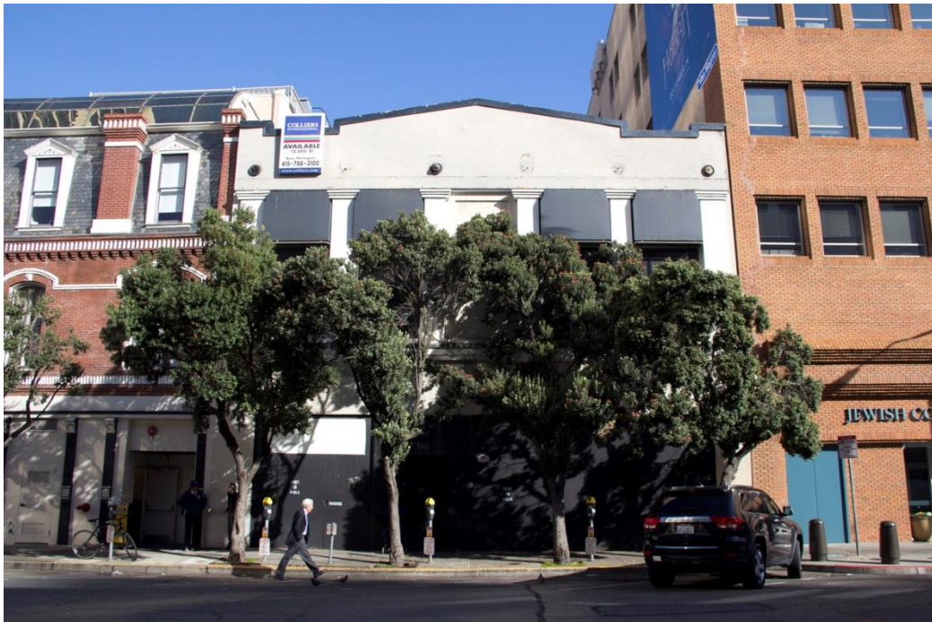
Existing façade facing Steuart Street:
