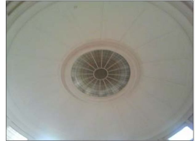
View of interior suspended ceiling above auditorium
