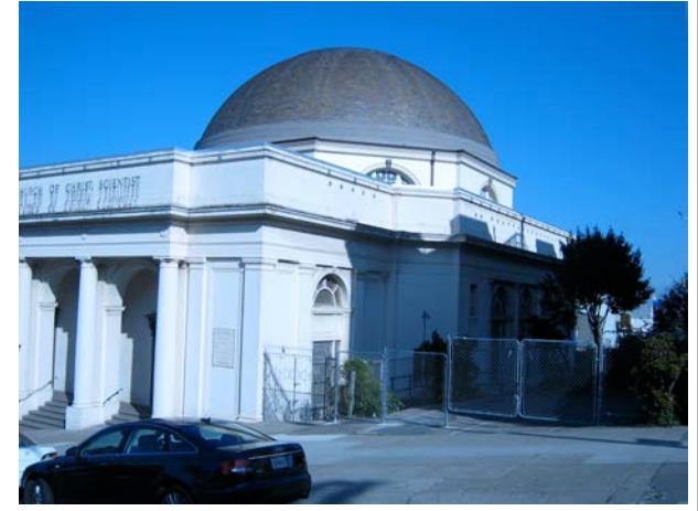
View of south and west facade from Dolores Street
