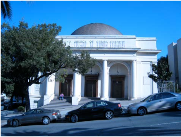
View of west facade from Dolores Street
