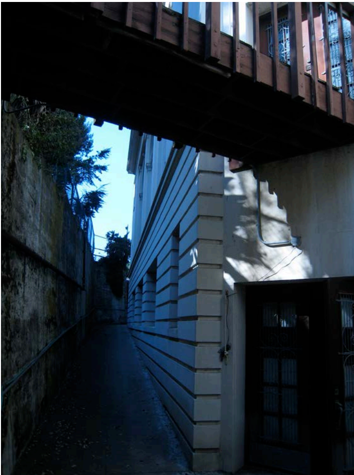
Western elevation lightwell view
