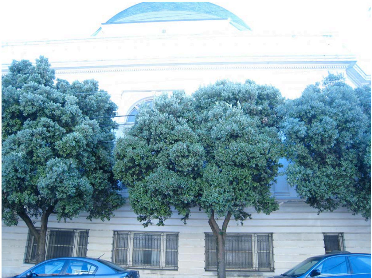
Building view, East elevation
