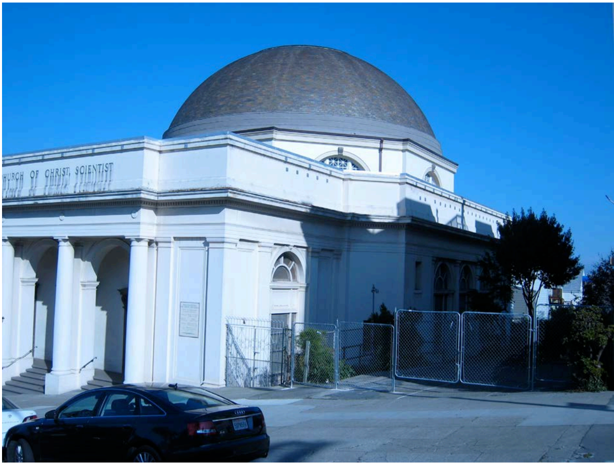
Building front and west elevation
