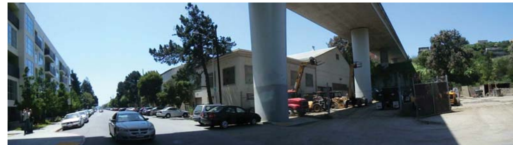
3 - LOOKING SOUTH - UNDER OVERPASS
