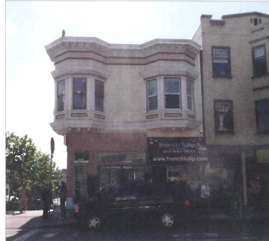
Photo 1 - View of entry & front facade from 24th Street
