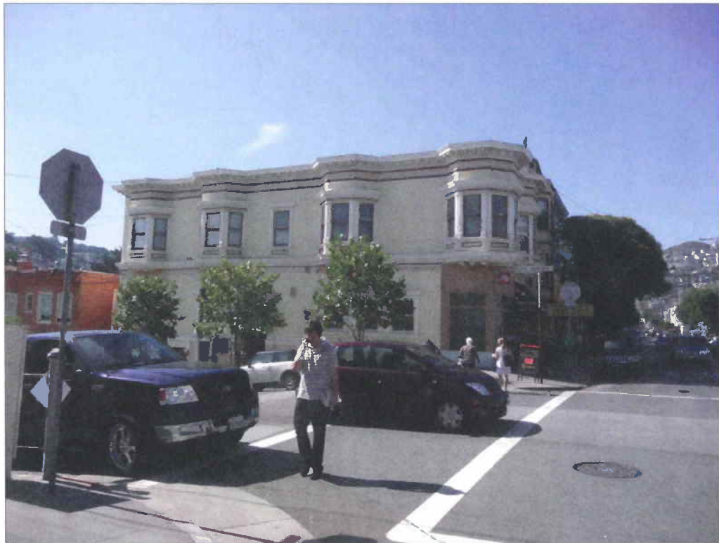
Photo 2 - View of side facade from Sanchez
