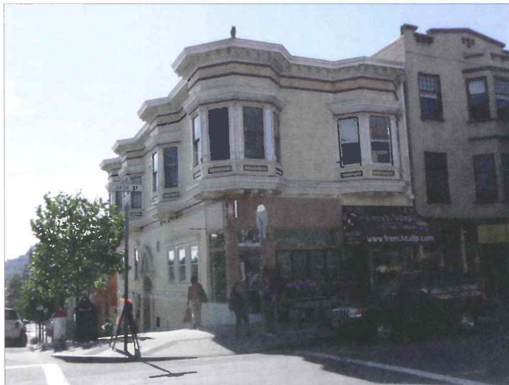
Photo 3 - View of south-west corner of 24th Street & Sanchez
